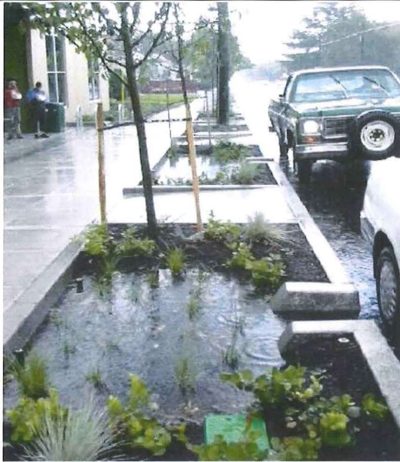
21. Portland, OR. Bioswale integrated between roadway and sidewalk.
