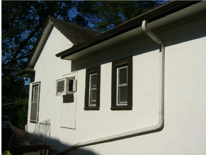
The side (south) façade showing second application of stucco cladding.
