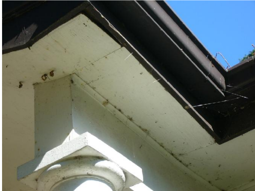
Architrave of plywood construction.
