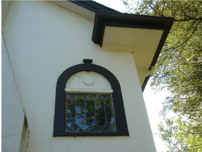
The side (north) façade at northwest corner with reconfigured 1960s window frame and original leaded comes.
