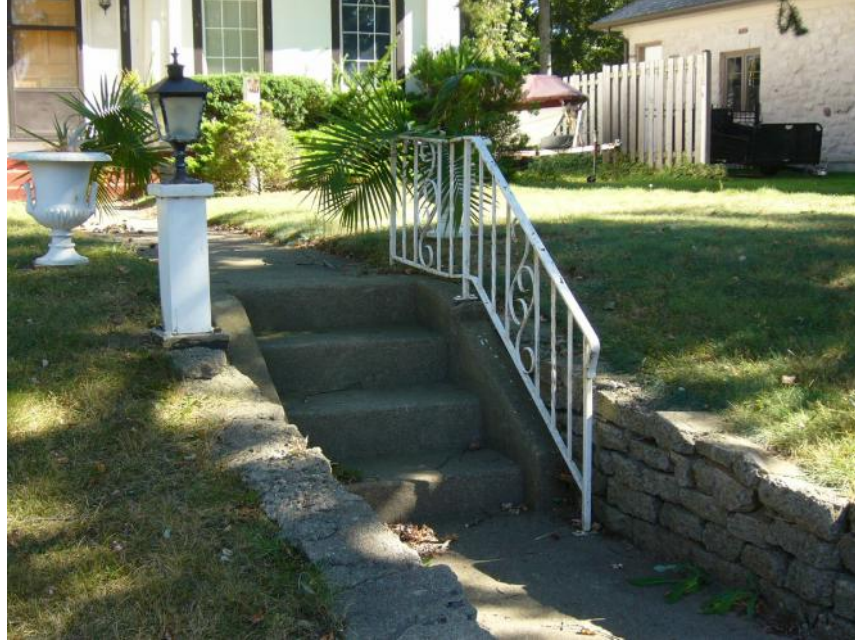
Cast-concrete steps with concrete rubble retaining walls to both sides.
