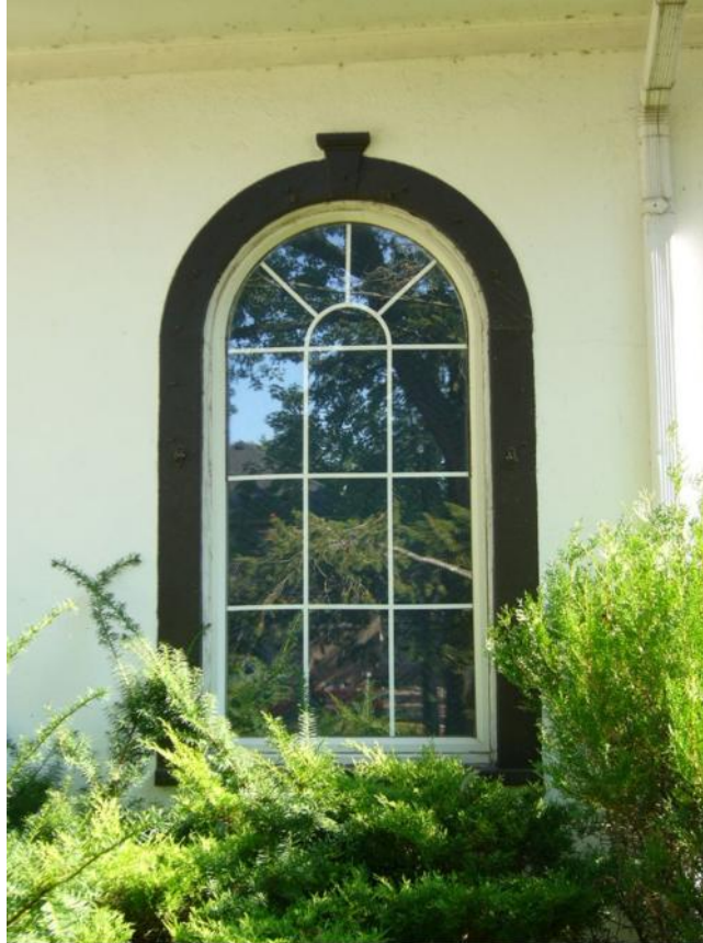
Original square headed windows transformed into round-headed windows of double-glazed units and synthetic muntins, surrounded by wood frame and lintel.
