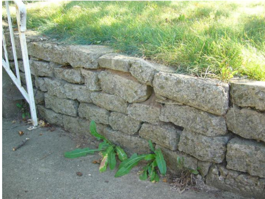
Detail of concrete rubble retaining wall.
