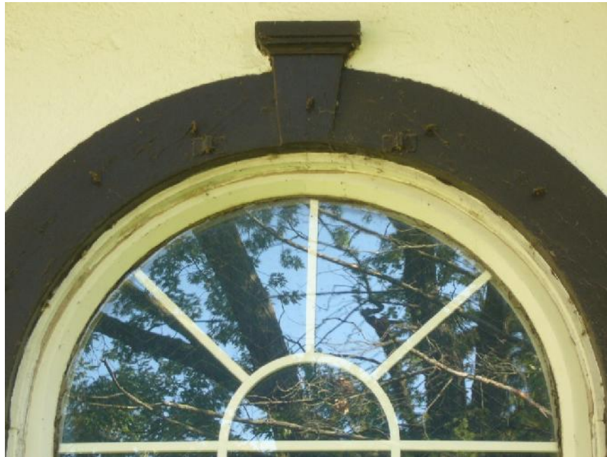
Detail of round-headed windows and synthetic muntins.
