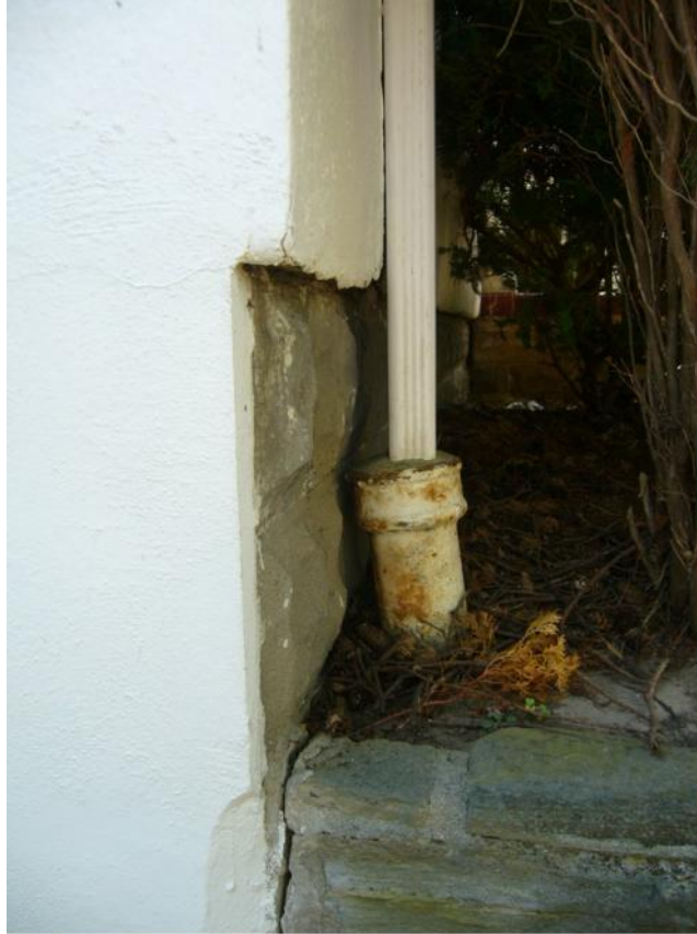
The front (west) façade at northwest corner showing extension of second application of stucco cladding hanging over the concrete block foundation.
