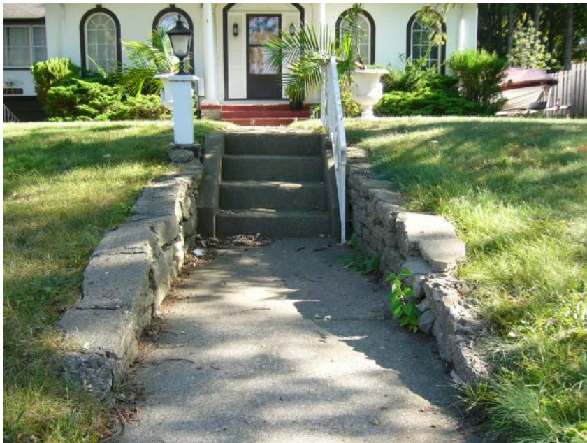
Concrete pathway and concrete steps with flanking coursed concrete rubble retaining wall.
