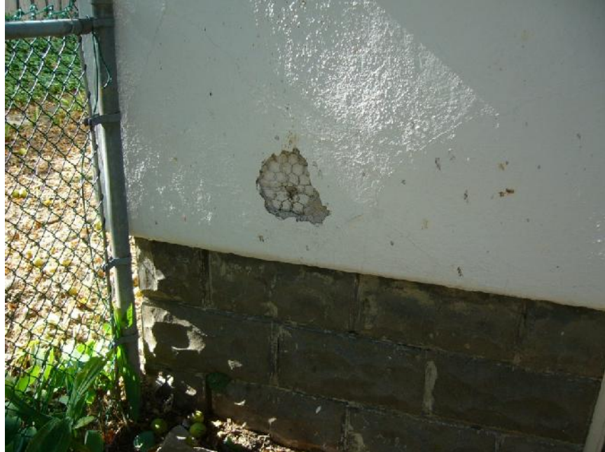
Southeast corner showing exposed layers of stucco, 1960 and 1920s.
