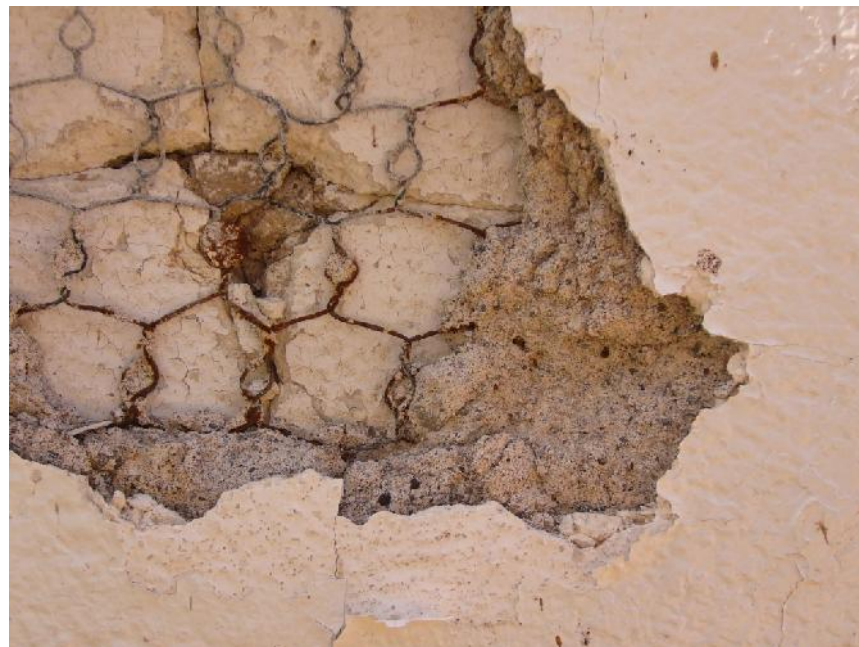
Detail of exposed layers of stucco, 1960 stucco and chicken wire mesh over deteriorated 1920s stucco.
