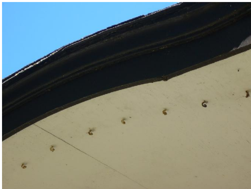
Plywood sheet in underside of porch roof.
