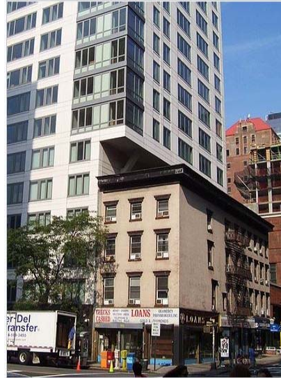
An example of air rights in use: a high-rise building extends over a four-story building in Manhattan
