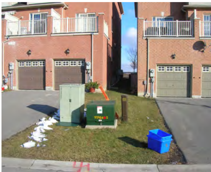
Fig. 6-61 to 6-62 (above) | Clustered plant is best located at the back side of a corner lot (top) rather than in between lots (bottom)
