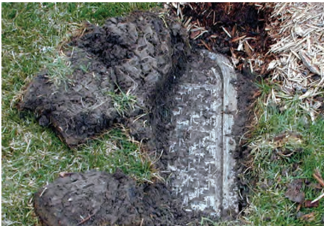
Fig. 5-3 | A FTG Handwell covered in sod by a homeowner, making it difficult to locate and access
