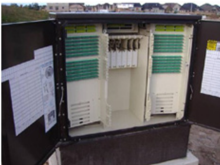
Example of an opened Central Splitting Point
