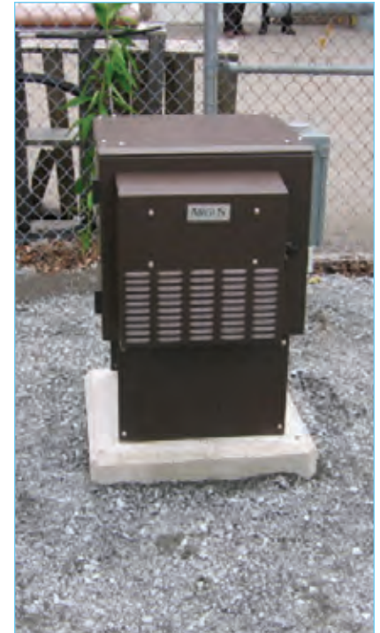
Fig. 4-15 | An Optical Network Unit appended to an Outside Plant Interface
