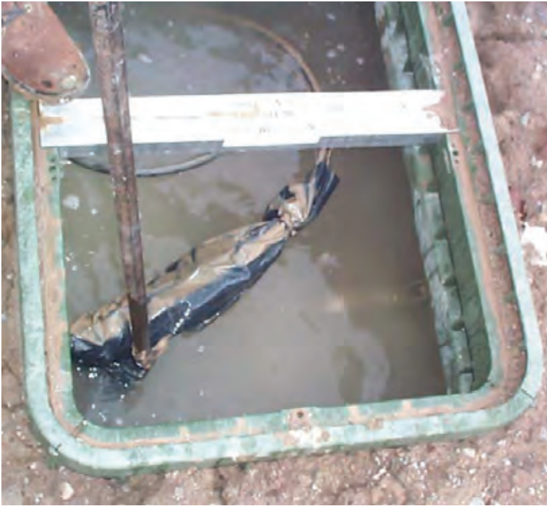
Fig. 5-1 | Extensive damage to a FTG Handwell caused by ice
