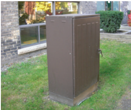
Example of a Fibre Distribution Interface
