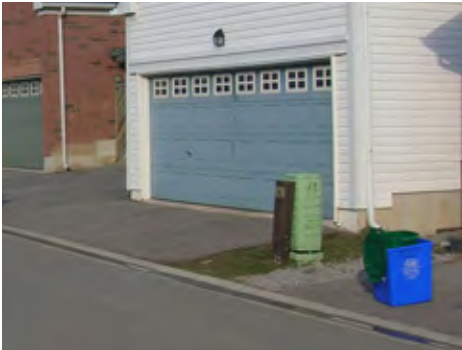
Fig. 6-57 (top) | Cabinet is best located at edge of green open space
