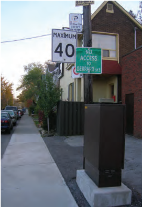
Fig. 6-15 | OPI cabinet located back from sidewalk and aligned with pole
