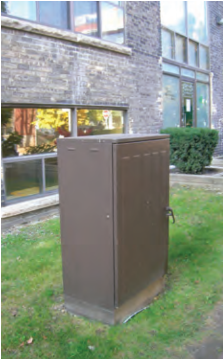
Fig. 4-14 | A Fibre Distribution Interface located in a reurbanized mixed-use area
