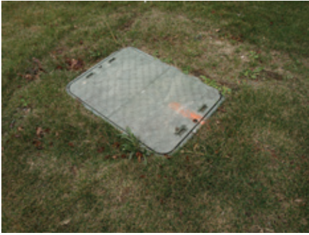
Example of a flush to grade handwell
