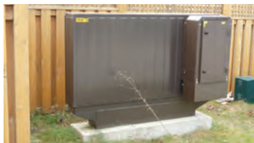
Fig. 4-7 to 4-8 | OPIs come in a variety of shapes and sizes depending on their vintage and locational context and may have modular additions
