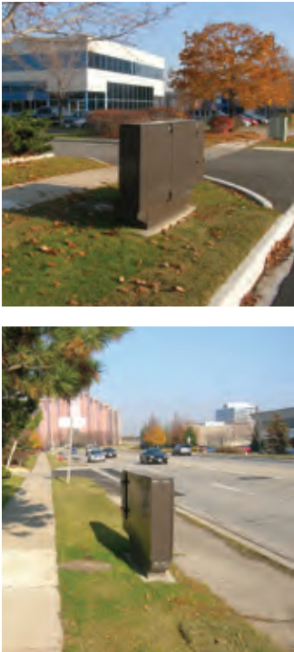
Fig. 6-47 to 6-48 | Well-located front boulevard cabinets; flush concrete base helps units blend in visually
