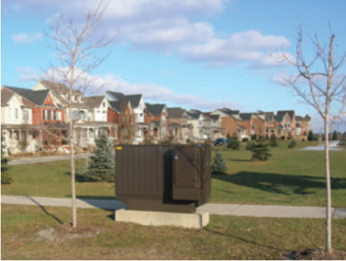
Example of a type of cabinet - in this case, an Outside Plant Interface (OPI)
