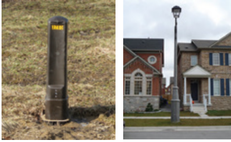
Example of a stand-alone servicing pedestal (left) and a pedestal integrated into a communication pole (right)
