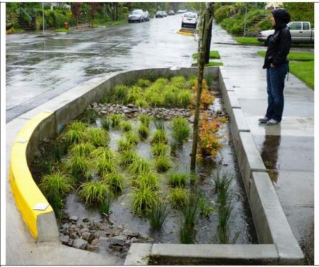
22. Portland, OR. Bioswale integrated between roadway and sidewalk.
