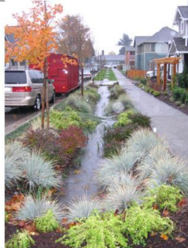
20. Portland, OR. Bioswale integrated between roadway and sidewalk.
