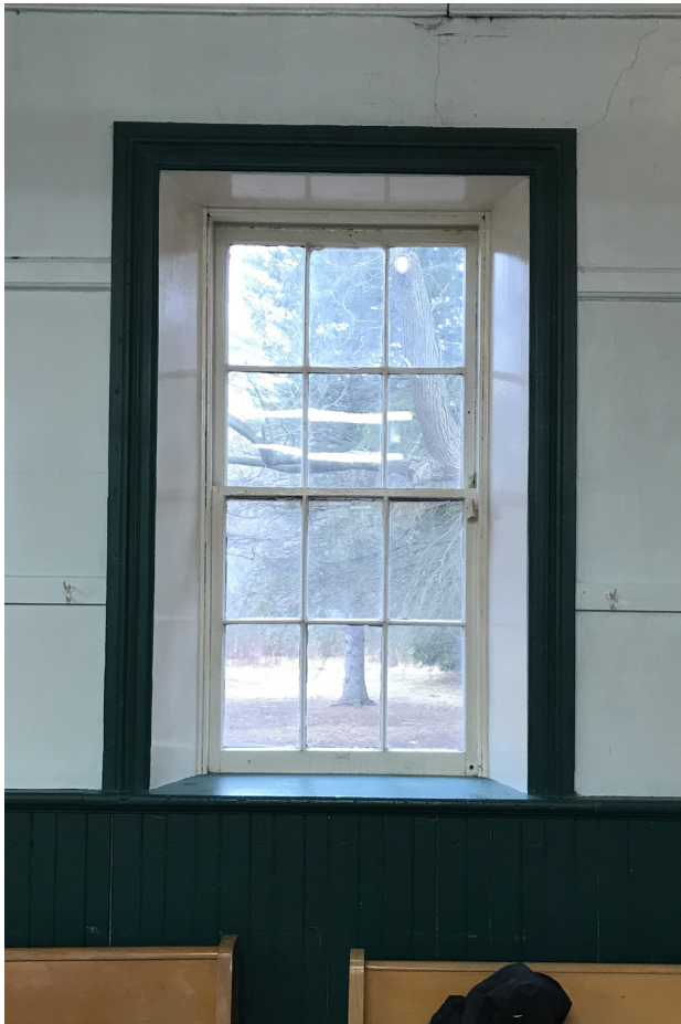
Original wood window, 6-over-6. Openings angle inward from interior side to exterior side of wall.
