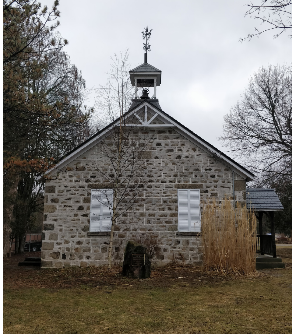
High pitched roof with gable ends.
