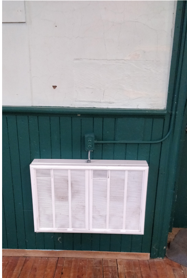
Heating by wall mounted radiators.
