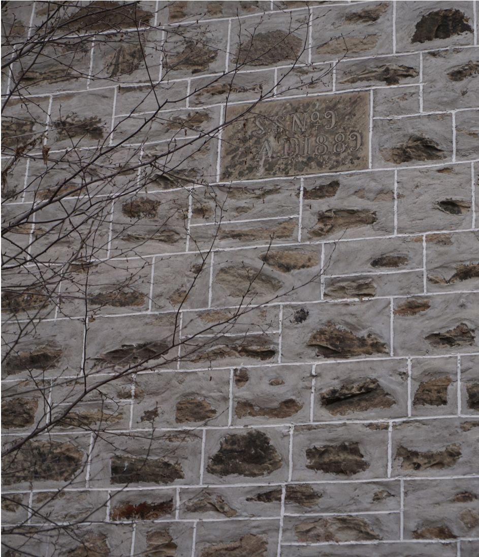
Stone cladding using local fieldstone (Mervyn Coulson Farm) and mortar made with sand from the Cleaver Mill Pond.
