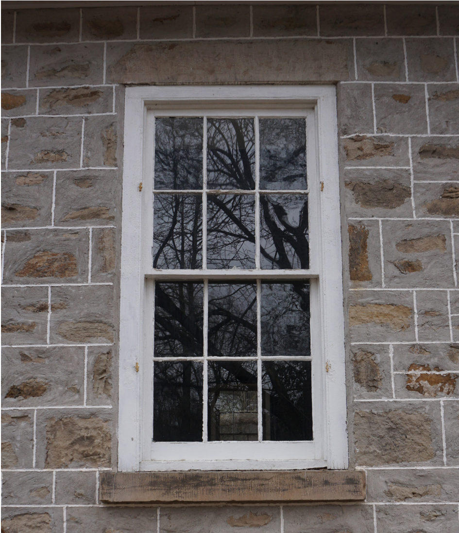
Example of windows (six-over-six panes) with stone sill and lintel
