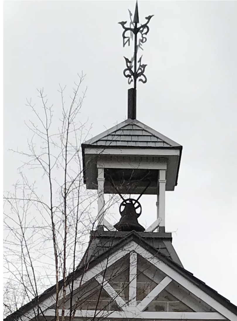
King post, bellcote, and weathervane
