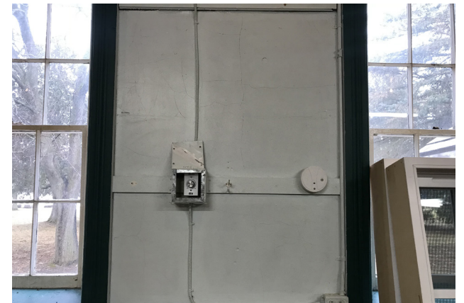
Damage to interior plaster work.
