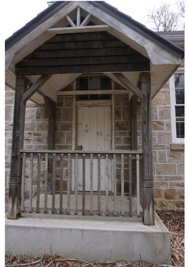
Main entrance on east side of building. Concrete steps and landing with wood frame porch enclosure.
