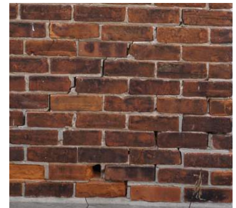
Examples of areas of masonry requiring crack repair and repointing over openings and near the corners of the house.
