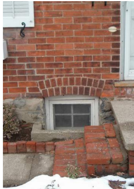
Arched brickwork over basement window.
