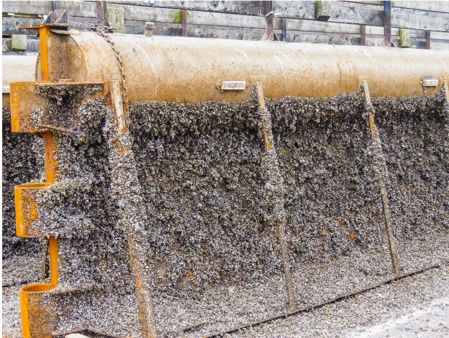
Current Wave Break Loaded with Shellfish(8/1/2016)
