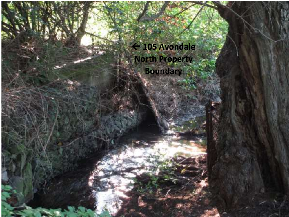
Collapsed Gabion Wall section at 105 Avondale (2014)
