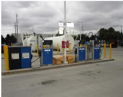
Refueling Pinch Point
