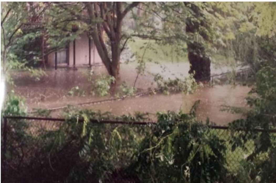
Creek – August 4, 2014 Looking from 105 Culvert toward 4342 BWP
