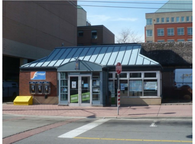
Downtown Burlington John Street Bus Terminal
