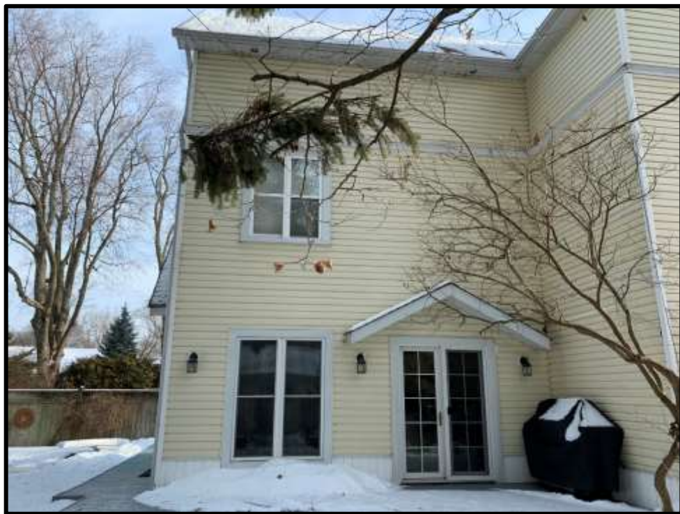
Image 16: West elevation of addition (Photo taken on January 22, 2020; Facing East)
