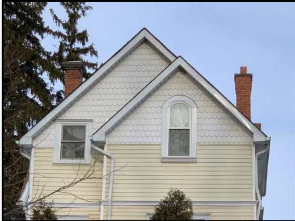
Image 3: Detail of front gable, window openings, fish scale shingles and red-brick chimneys (Photo taken on January 22, 2020; Facing Northeast)
