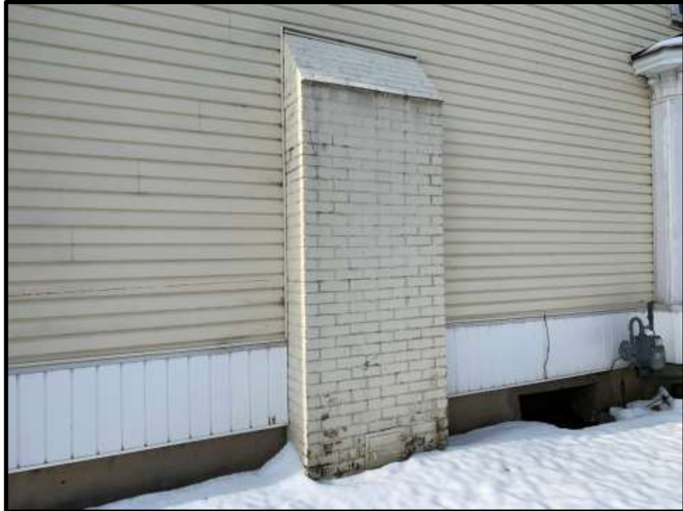
Image 21: East elevation detail of painted brick chimney (Photo taken on January 22, 2020)
