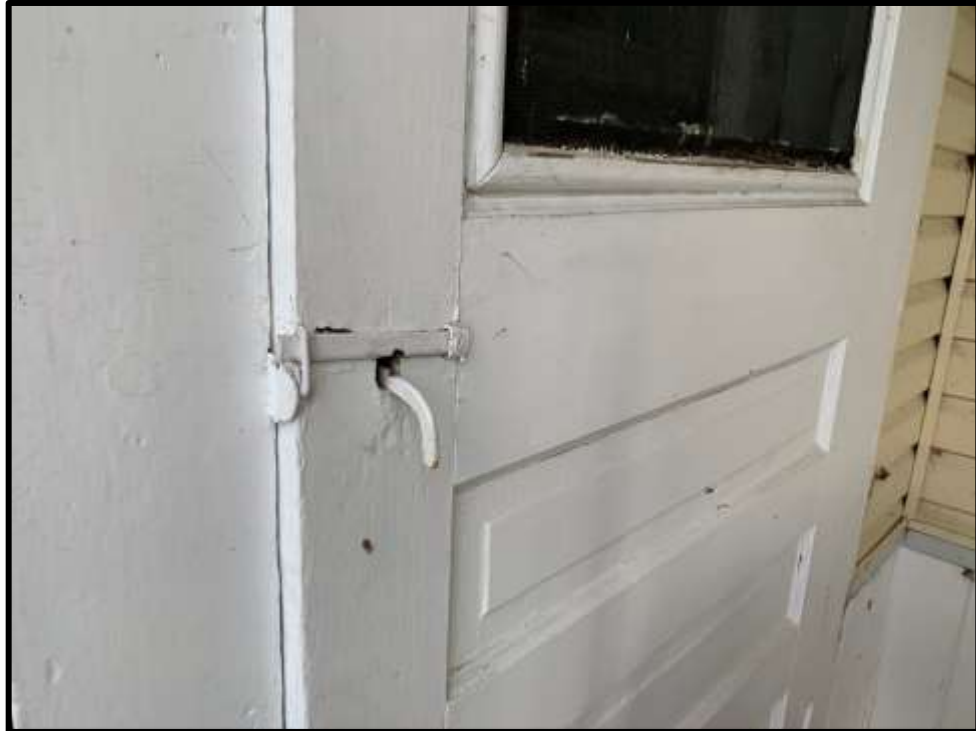
Image 13: Detail of door latch in doors under porch in west and south elevations (Photo taken on January 22, 2020)
