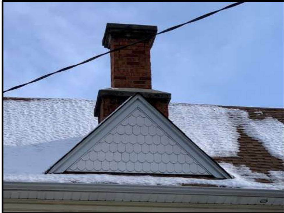
Image 15: Chimney at west elevation (Photo taken on January 22, 2020; Facing East)
