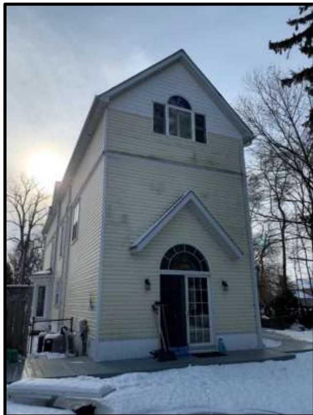
Image 18: Northeast corner and north elevation (addition) (Photo taken on January 22, 2020; Facing Southwest)
