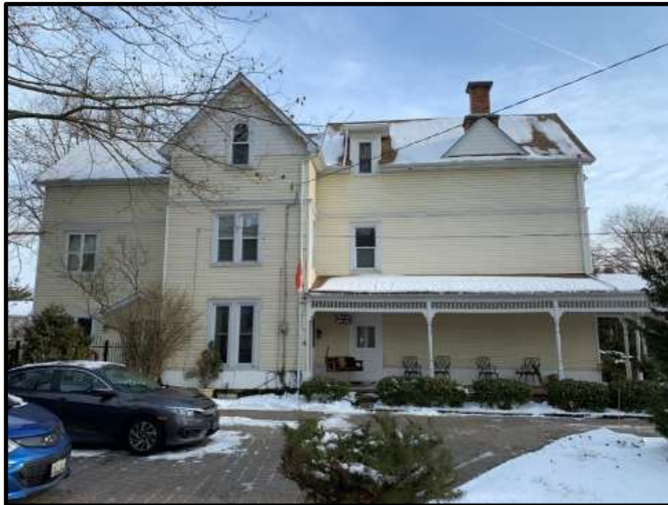
Image 10: West elevation (Photo taken on January 22, 2020; Facing East)
