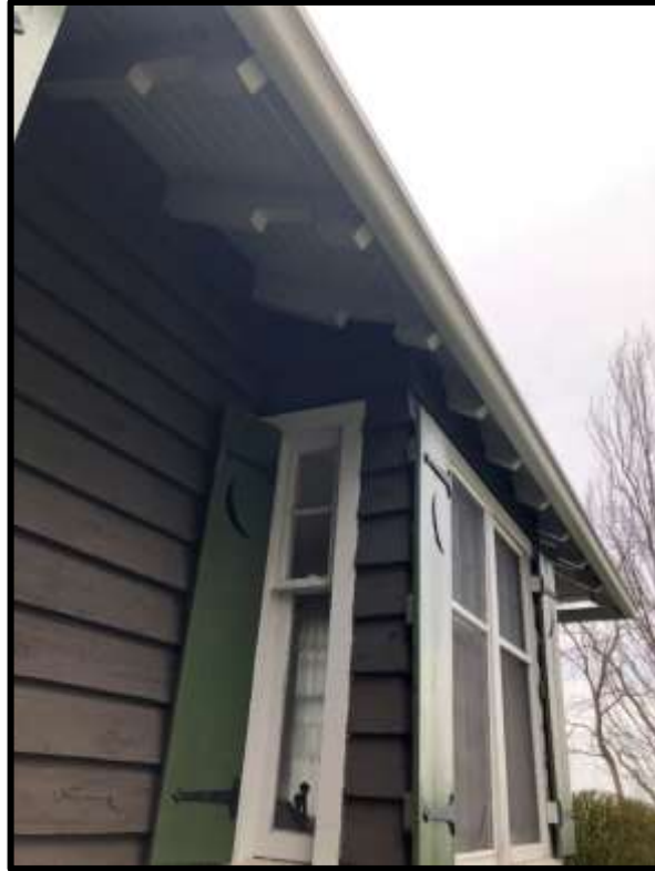
Image 19: Detail of Rafter Tails, Clapboard Siding and Bay Windows on West Elevation (Photo Provided by Client; Taken on April 29, 2020)
