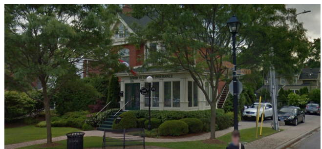
Office entrance directly accessible from Brant Street
