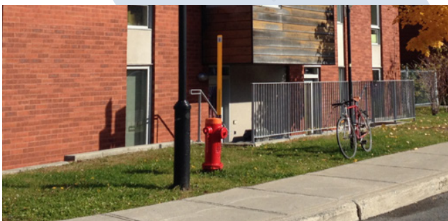
Above ground utilities should not be placed in the Clear Path Zone
