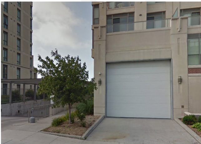
Service area integrated into the building design
