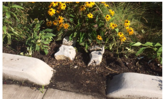
Rain gardens help to increase the infiltration of stormwater
