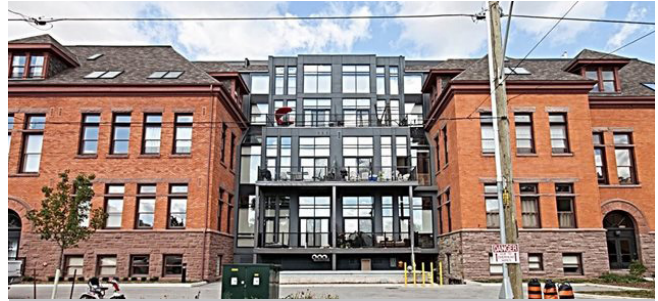
Adaptive use and preservation of Cultural Heritage Buildings
