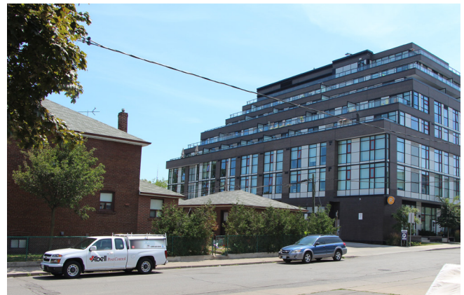
Terraces used to accommodate the transition from low to mid rise buildings
