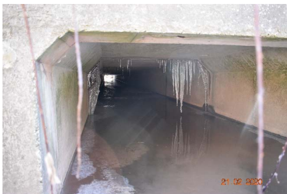
Photo WH.15: Barrel View Looking South Towards Outlet, Note Drainage Through Joints
