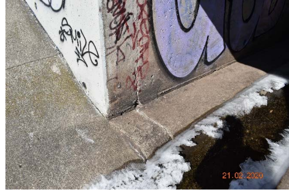
Photo F.16: Medium to Wide Cracking at Culvert Outlet
