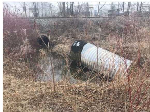
Photo ER.6: East Rambo FCF inlet from north, note scour repair required
