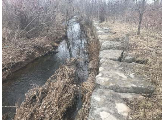
Photo ER.10: creek u/s of East Rambo FCF inlet in west corner – minimal scouring
