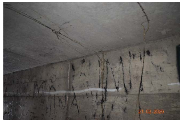
Photo F.18: Stalactites Along Barrel Soffit and Culvert Walls
