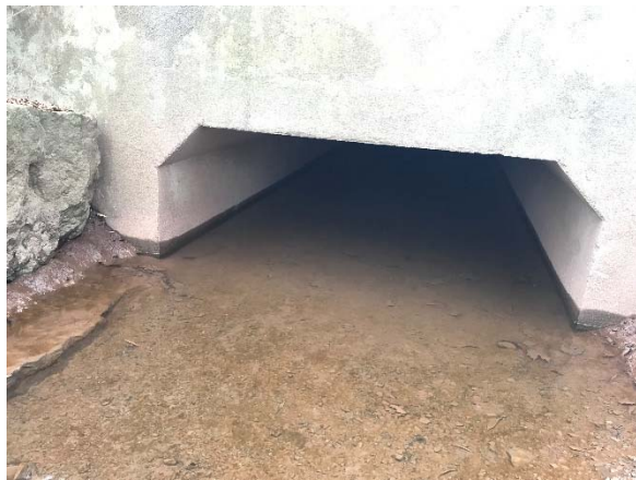
Photo WH.9: Downstream face of outlet control culvert, note sediment deposition mid-depth
