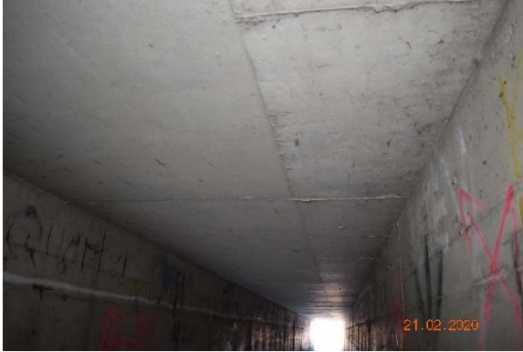
Photo F.15: Typical Condition of Barrel Soffit
