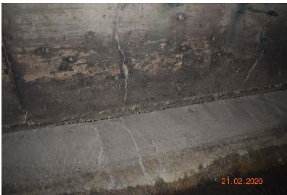
Photo F.17: Segregation of Concrete Below High-Water Level
