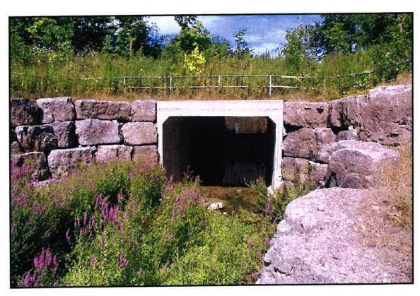
Photo 9.3 - Looking upstream towards the culvert and cut-off wall structure
