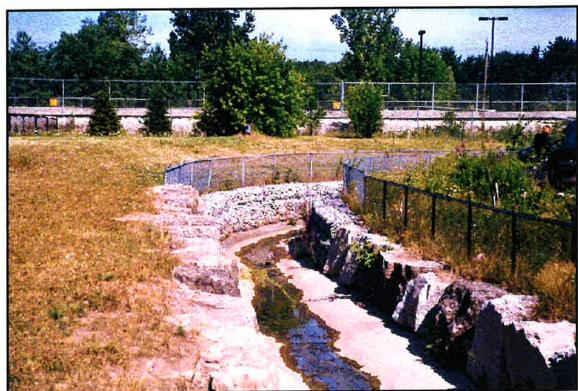
Photo 3.1 Looking upstream at the transition from the vertical gabion walled channel to the armour stone lined channel from station 0+020.
