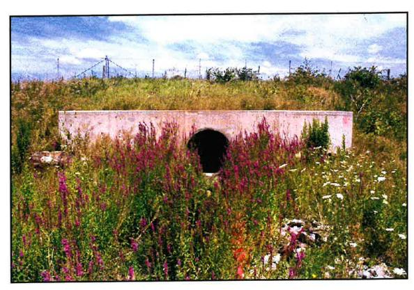
**Photo 7.7** - Downstream face of the 1350 mm concrete pipe extending for 32 metres under the 403 west to Brant Street north/south ramp, at the northeast corner of the site.
