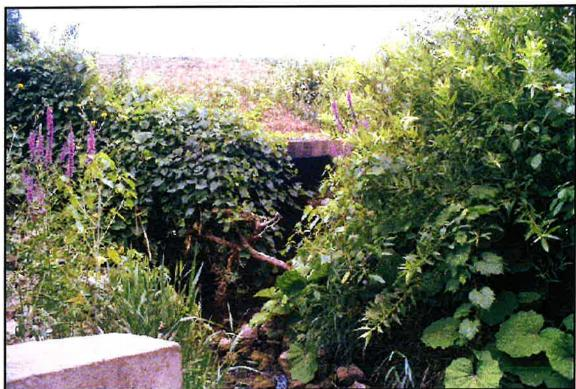
Photo 10.1 - View of the upstream side of the culvert crossing under the North Service Road. Note the debris blocking the culvert opening.
