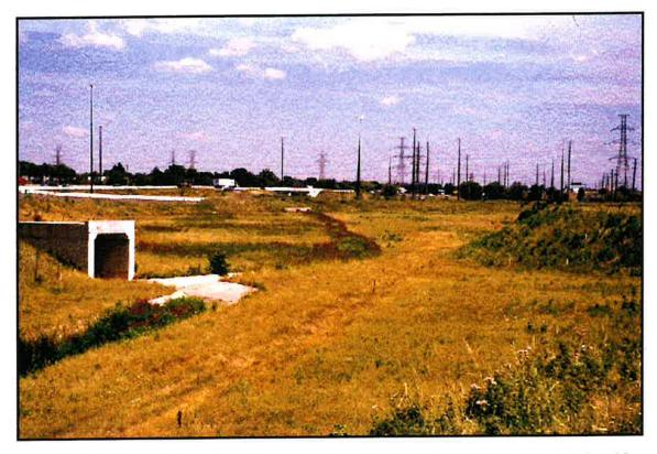
Photo 7.5 - Looking upstream at the pond from from the previous location atop the berm, with the 5.05 x 5.05 metre culvert on the left and the 1350 mm culvert in the centre.
