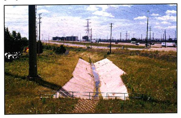
Photo 6.4 - Looking downstream at the concrete to terrafix block channel transition from the top of berm above the outlet culvert.
