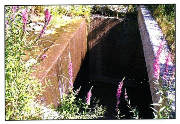
Photo 9.5 - Looking down into the cut-off wall structure at the upstream limit of the works
