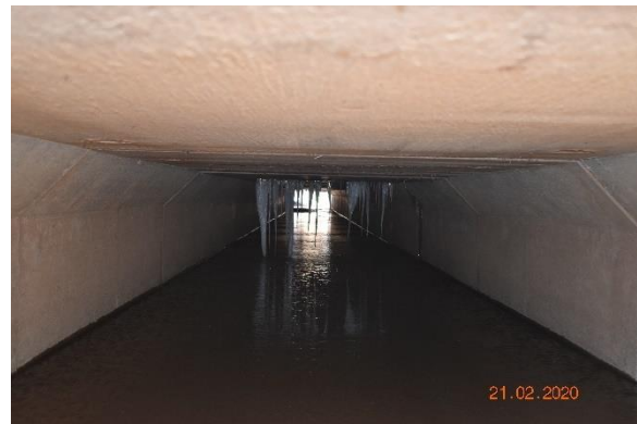
Photo WH.14: Barrel View Looking North Towards Culvert Inlet, Note Drainage Through Joints
