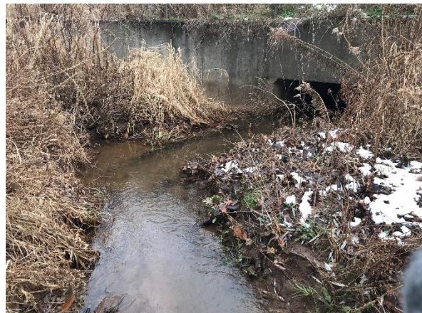
Photo WH.10: Channel immediately upstream of outlet control culvert, minor erosion, deposition in culvert
