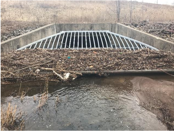
Photo ER.9: East Rambo Facility outlet control culvert with safety grate and debris
