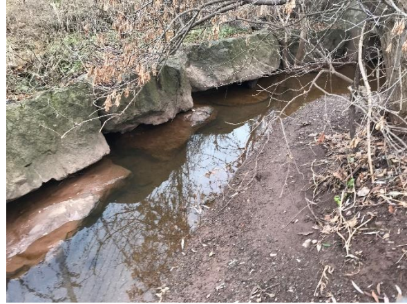
Photo WH.8: Immediately downstream of outlet culvert – armour stones potentially undermining
