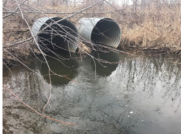
Photo ER.8: East Rambo FCF d/s end of twin inlet culverts to main Facility at west end
