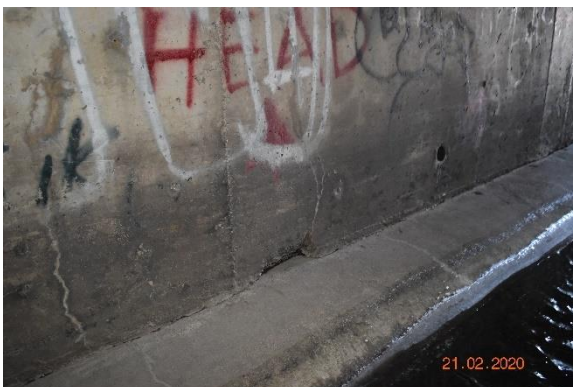
Photo F.19: Localized Spalling with Exposed Rebar at Culvert Wall
