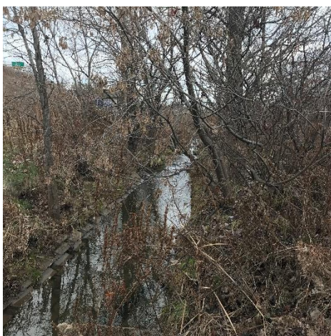
Photo F.5: Lined channel in lower section, near inlet, note woody vegetation
