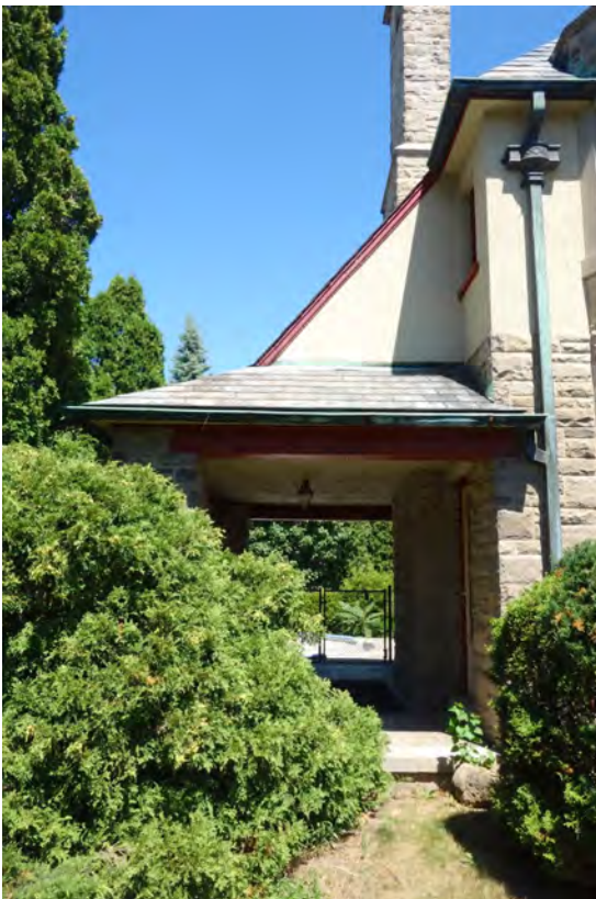
MAIN ELEVATION – HIGH SLOPED ROOF – INTEGRATED PORCH – TALL CHIMNEY – COPPER GUTTERS & DOWNSPOUTS TO CISTERN
