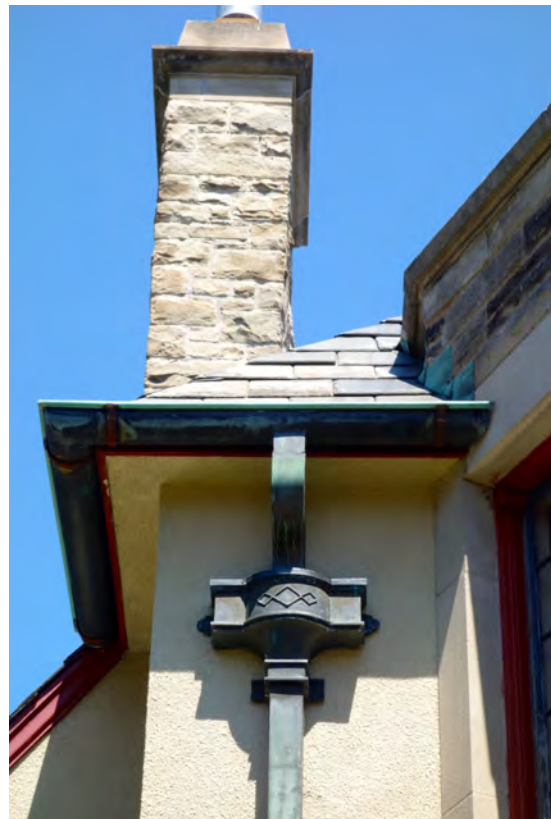
MAIN ELEVATION – HIGH SLOPED ROOF – INTEGRATED PORCH – TALL CHIMNEY – COPPER GUTTERS & DOWNSPOUTS TO CISTERN
