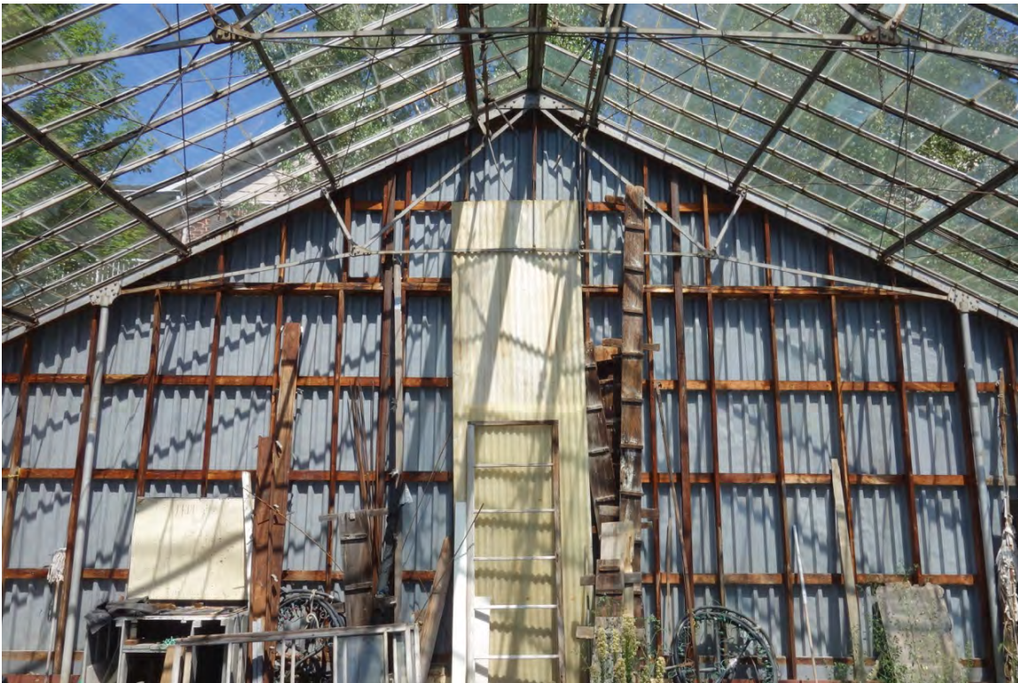
GREENHOUSE INTERIOR - METAL FRAMING - GLAZING ON 3 SIDES AND CORRUGATED METAL ON THE REAR ELEVATION
