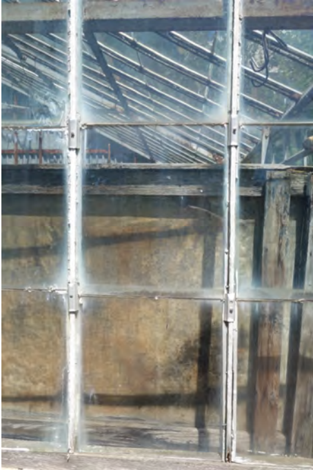
FIXED GLAZING WITH METAL CLIPS
