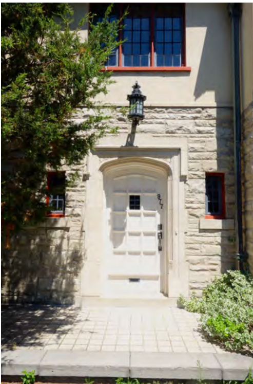
MAIN ELEVATION - CUT STONE, STUCCO & CAST STONE – SLATE ROOF W. COPPER FLASHINGS WOOD PANELED DOOR – STEEL CASEMENT WINDOWS
