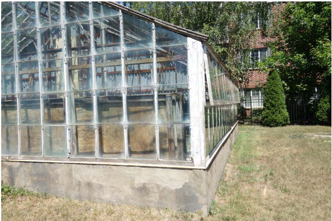
GREENHOUSE – FIXED GLAZING ON THE FRONT ELEVATION & OPERABLE WOOD SASH ON THE SIDE ELEVATION
