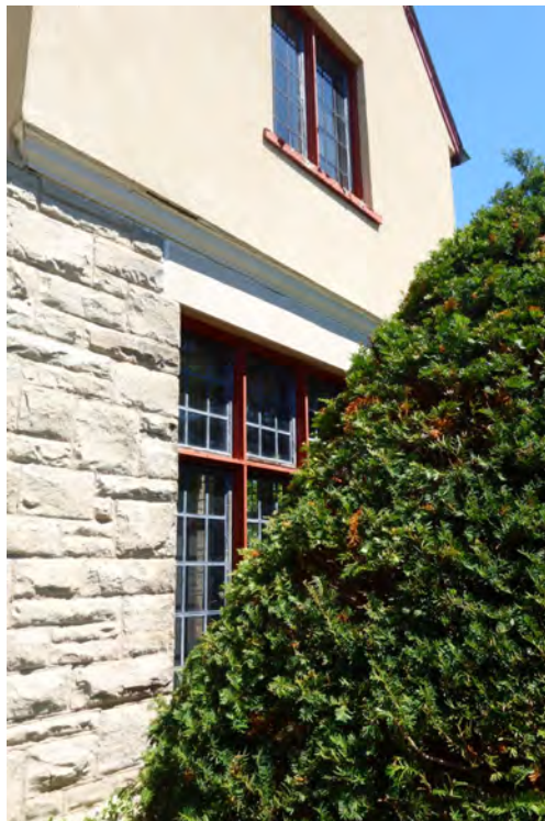
MAIN ELEVATION - CUT STONE, STUCCO & CAST STONE – SLATE ROOF W. COPPER FLASHINGS WOOD PANELED DOOR – STEEL CASEMENT WINDOWS
