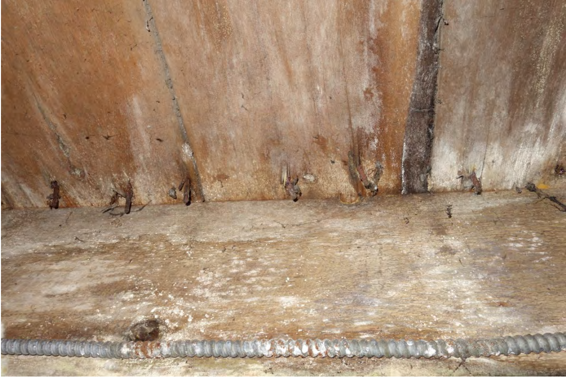
FLOOR FRAMING BELOW BACK PART – square nails
