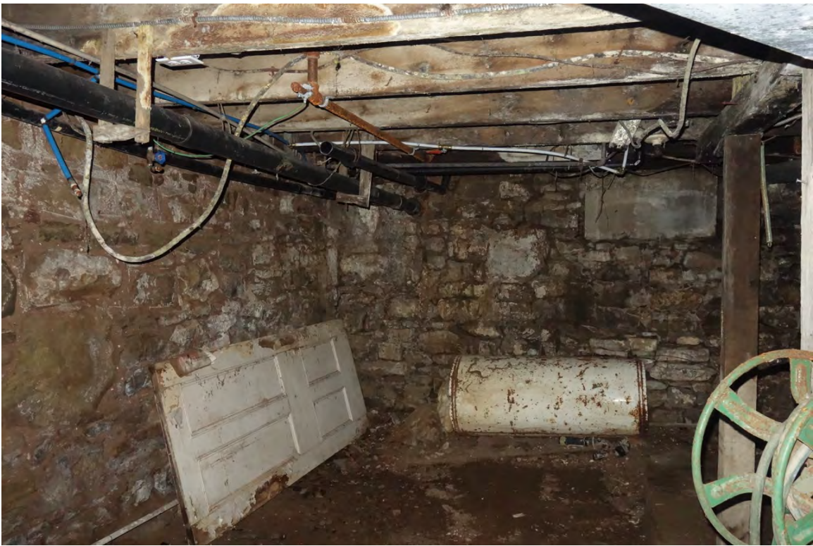
BASEMENT & RUBBLE STONE FOUNDATION BELOW BACK PART
