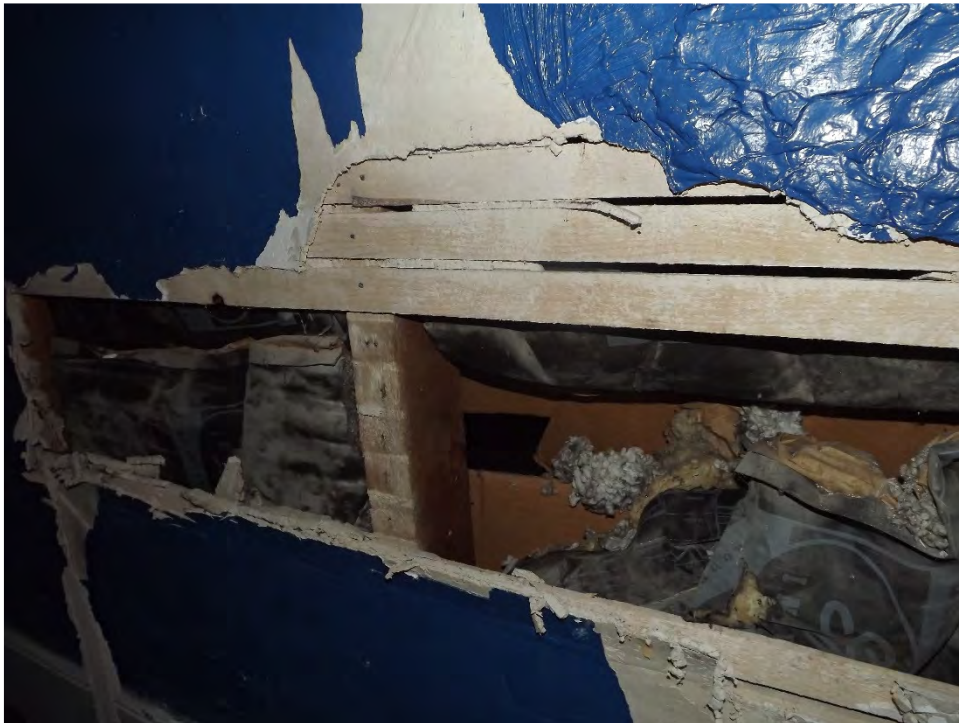
Circular sawn lath and framing in the rear wing
