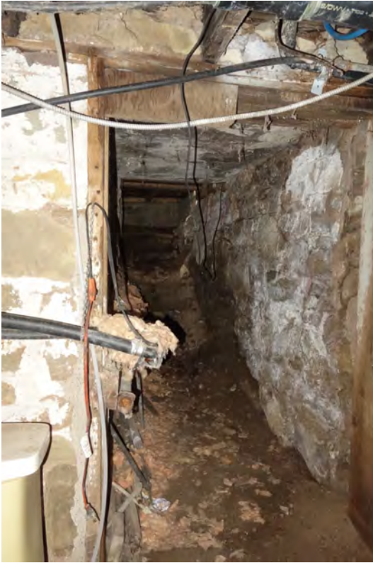
CRAWL SPACE & HALLWAY BELOW THE FRONT PART – very thick wall between front & back
