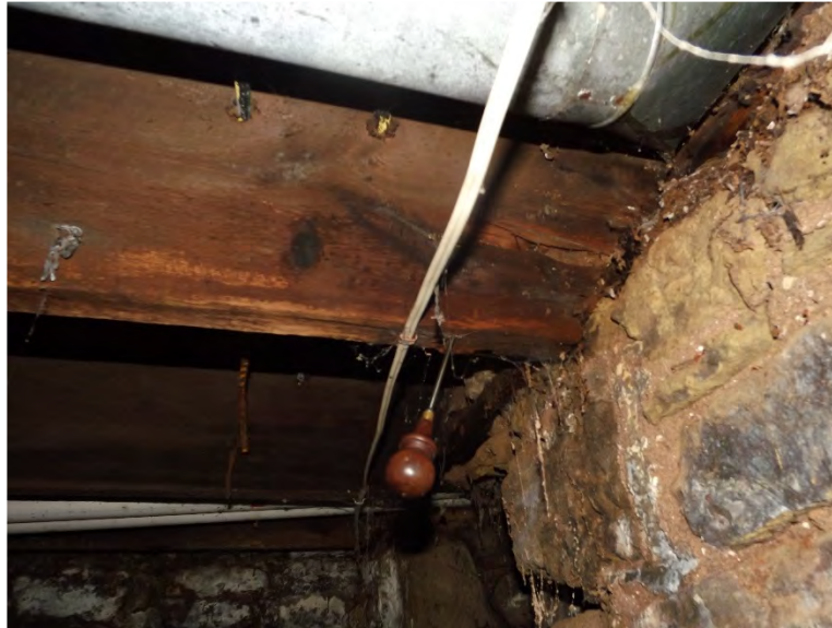
Damp wall, rotten plate, and awl inserted 2" into joist
