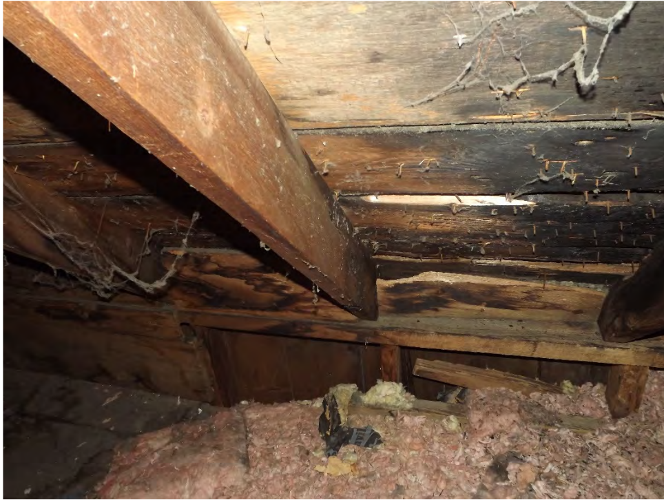
Balloon framing and circular sawn lumber; note the charring from a fire
