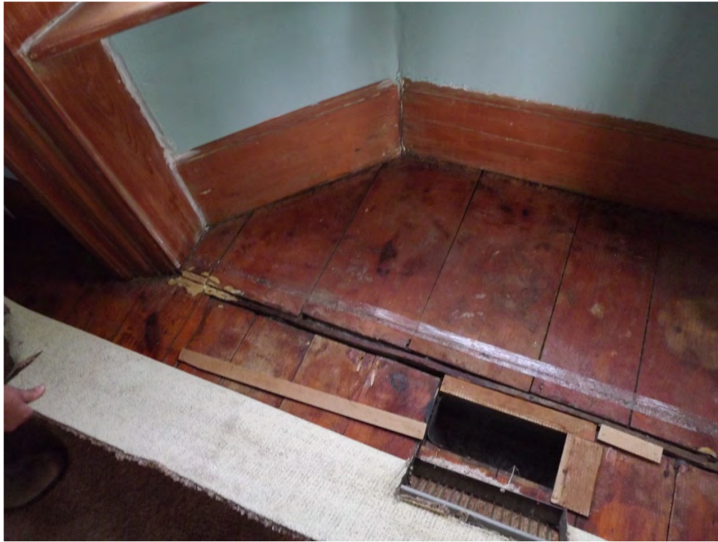
Bay window floor showing poor connection
