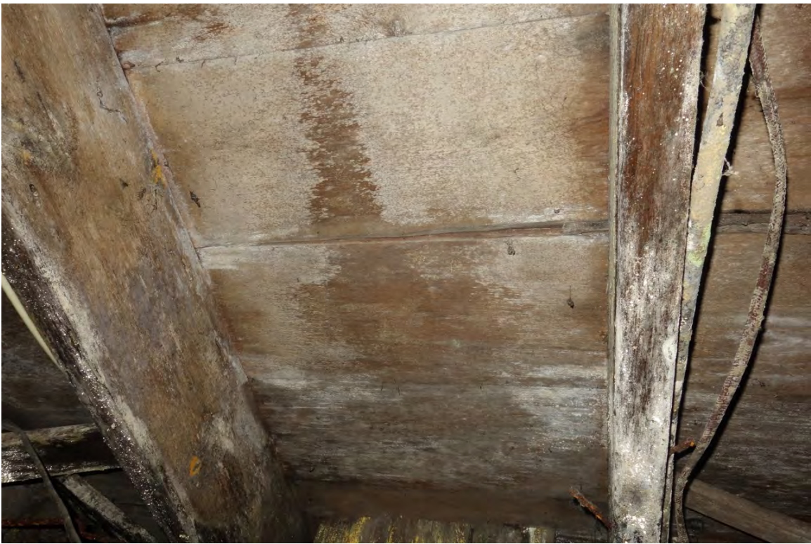
FLOOR FRAMING BELOW BACK PART – wide boards
