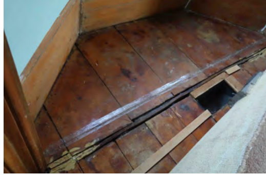
FRONT PARLOUR - there is a substantial gap in the flooring at the bay windows that is evidence of alteration and poor workmanship (right)
