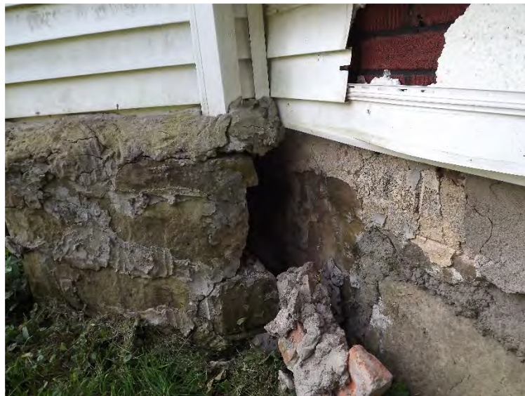
Bay window foundation and later repairs have failed
