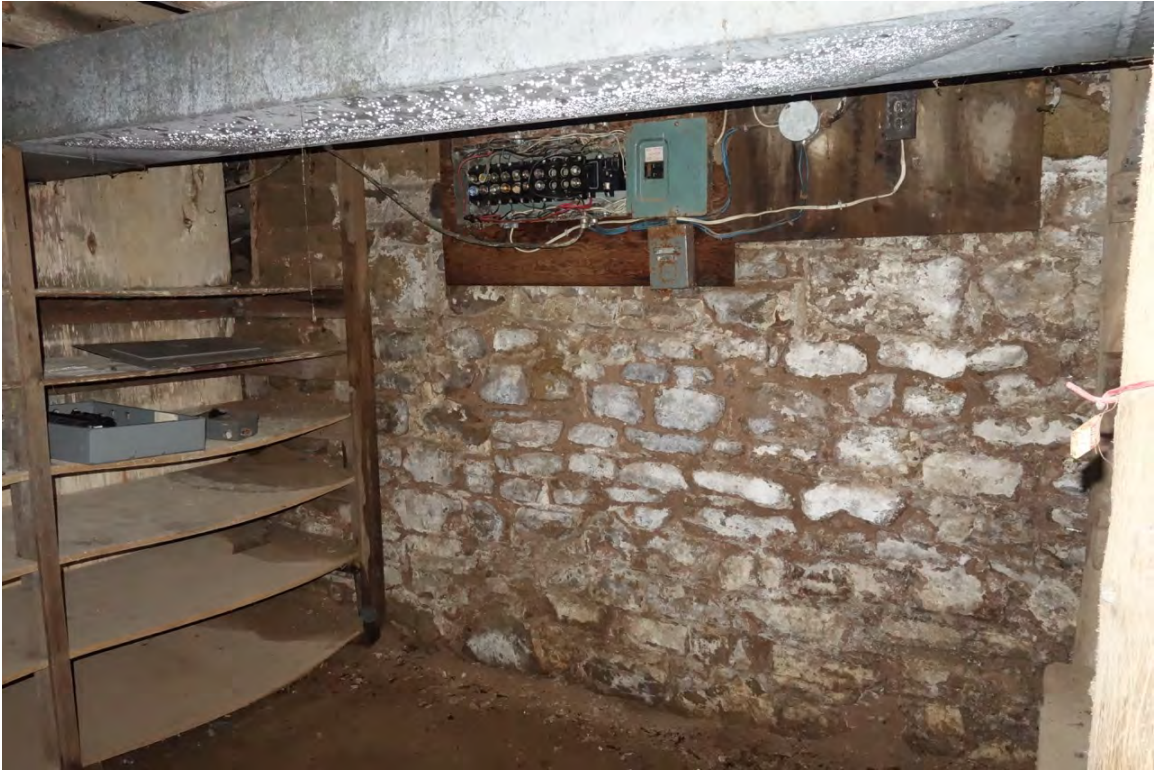
BASEMENT & RUBBLE STONE FOUNDATION BELOW BACK PART
