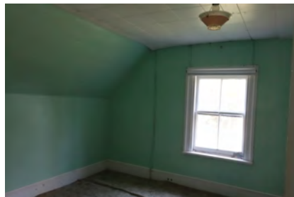
TRANSITION – there is a level change at the top of the stair landing that evidence of alteration and poor workmanship (left) – modern ceiling tiles in the bedroom is evidence of condition issues (right)
