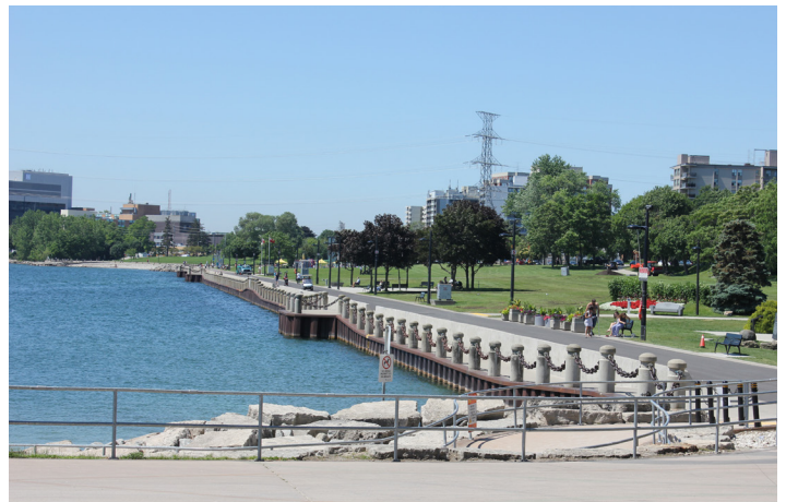
Looking west toward Spencer Smith Park (South and West)
