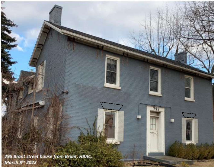
Flat arches visible beneath paint
