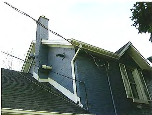
Exhaust vents and later chimney addition.
