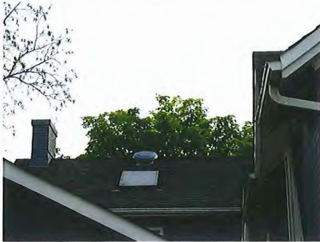
Skylight and roof vent.
