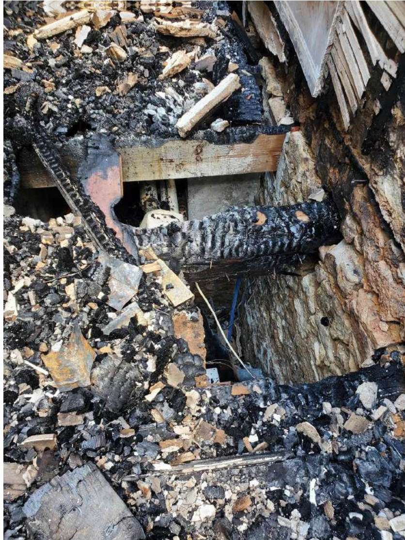
Figure 1: Typical Condition of Interior Ground Floor Framing (Over Basement) on South 2/3 of Building
