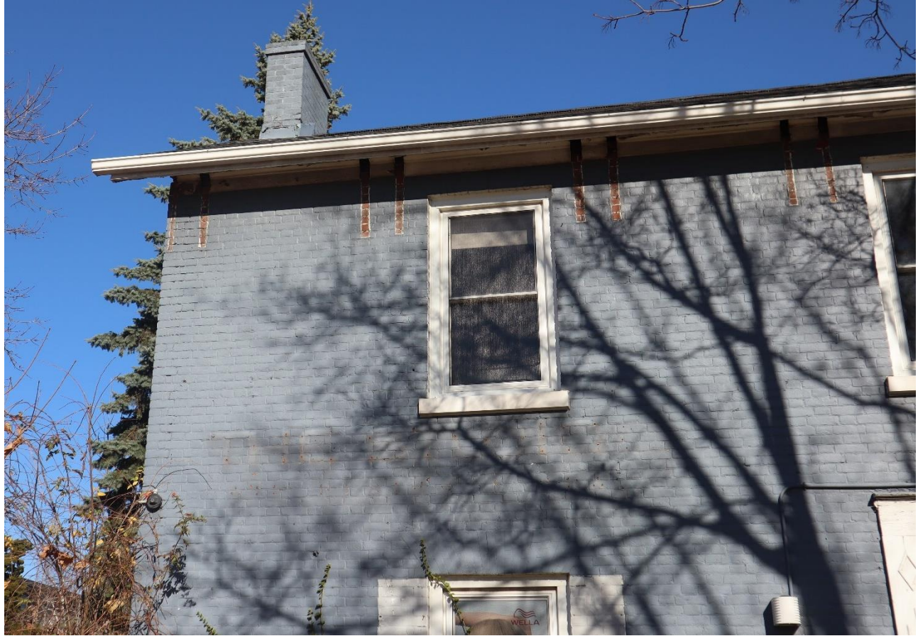
Photograph 8: View of the front façade (west elevation) of the original house, showing the former location of the paired cornice brackets (AECOM, November 2022)
