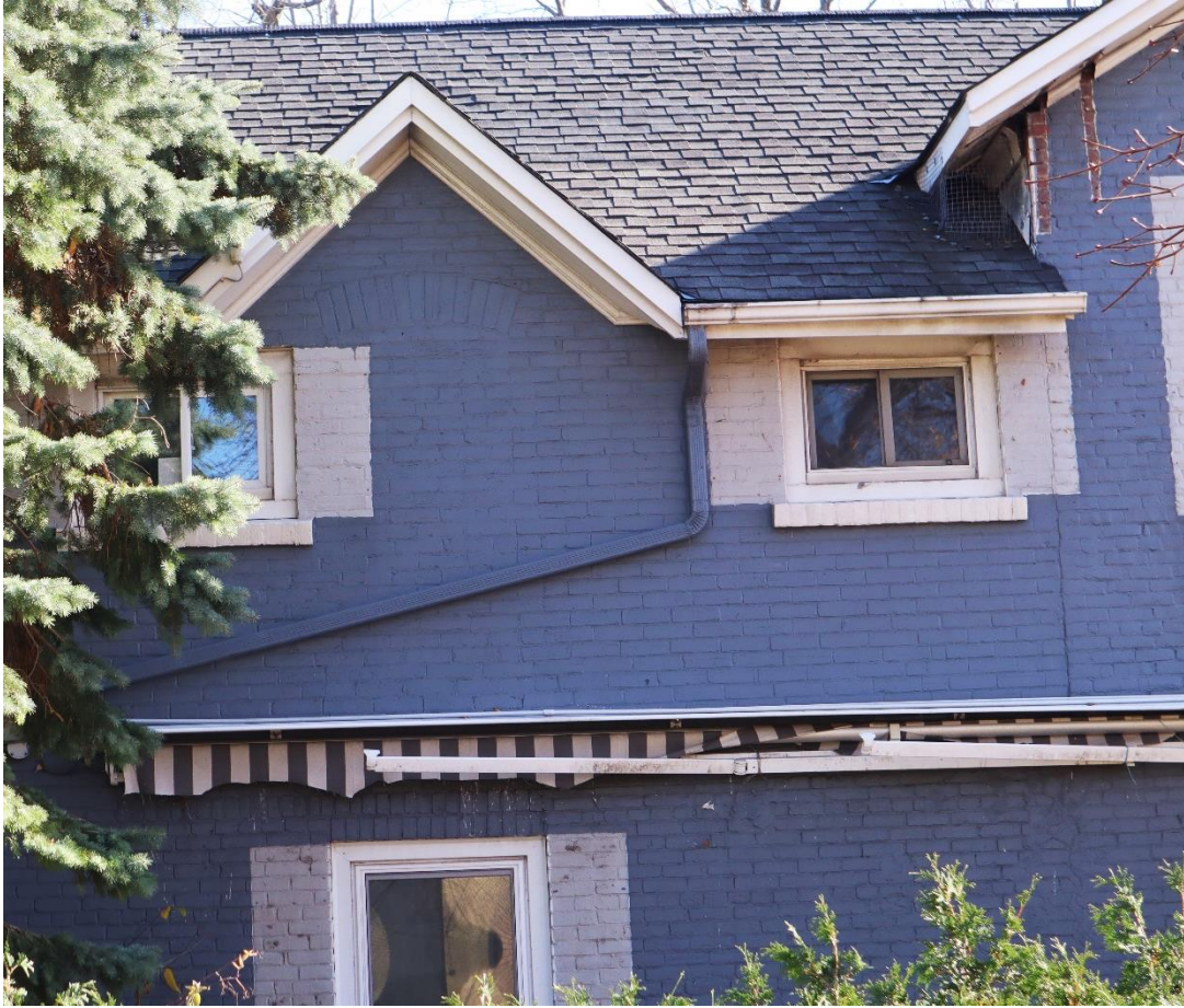
Photograph 12: View of the north elevation of the two-storey addition (Addition 1), showing former gable window opening with segmentally arched brick voussoirs and the second storey construction joint (AECOM, October 2022)
