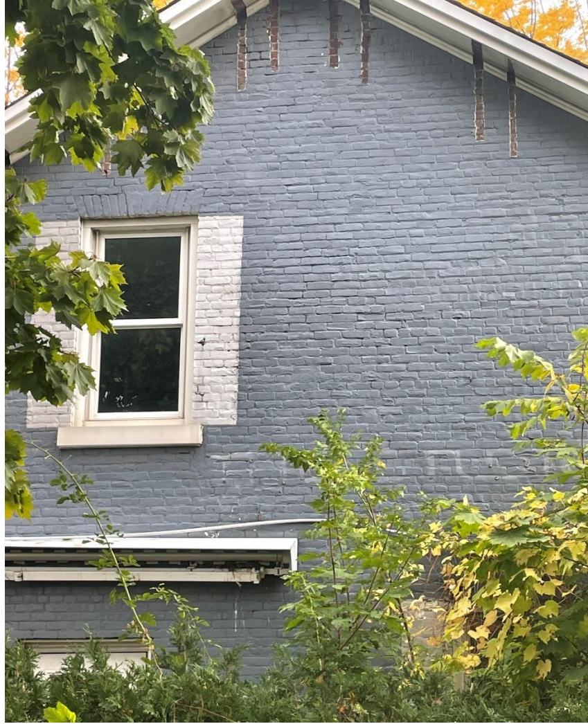
Photograph 13: View of the north elevation of the original house, showing the brickwork and jack-arched brick voussoirs of the second storey above the window (AECOM, October 2022)
