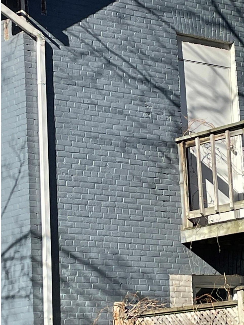
Photograph 11: Close-up of the south elevation of the original house, showing the common bond brickwork (AECOM, November 2022)
