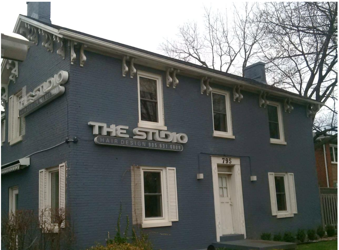
Image 6: Façade in 2015 with painted brick, metal shutter added to the ground floor, and the paired wood brackets (City of Burlington, 2015)
