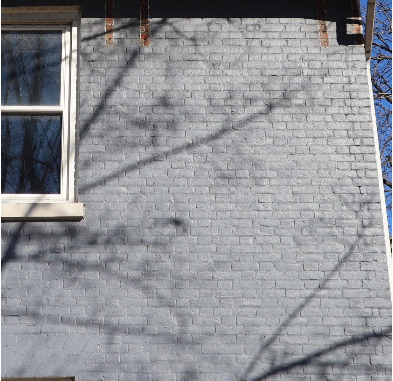
Photograph 9: Close-up of the façade (west elevation) of the original house, showing the Flemish Bond brickwork (AECOM, November 2022)
