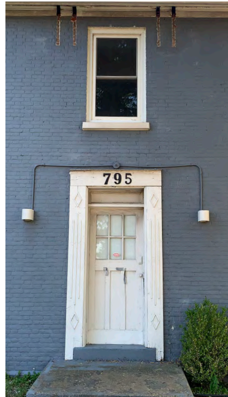
View of West Elevation of missing brackets, typical window and existing door that is not original to the building. Source: ATA Architects Inc (2022)
