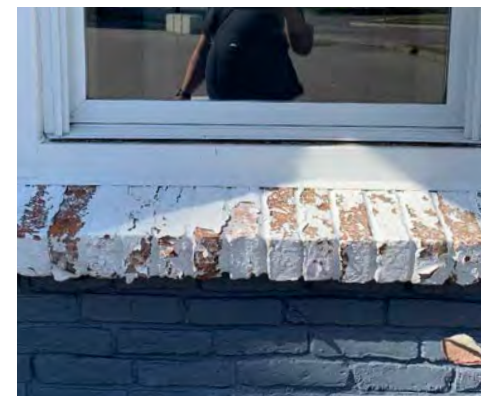
View of the South Elevation and typical brick sill not original to the house Source: ATA Architects Inc (2022)
