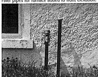
The stone façade and stone sill with the windows are visible due to the deterioration of the stucco. Modern aluminum storms have been installed over the wood windows.
