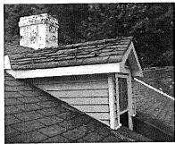
Aluminum soffit and eaves troughs have been added. The stucco is failing where the wall meets the roof, such damage is common on all foresdes.
