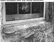
Stone detailing is still visible along the corners of the original front portion of the house. Typical damage to the lower portions of the stucco near grade.
