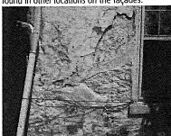
Stucco is deteriorating and the foundation is exposed. This situation is most prevalent on the west façade and is present to a lesser degree on others.
