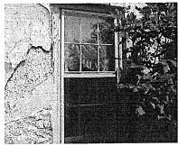
Poorly patched crack in exterior wall at the northwest corner, similar situations can be found in other locations on the façades.
