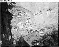
The mortar is deteriorating and breaking up. Damage is most prevalent on the west facade but occurs to a lesser extent on the other faç ades.
