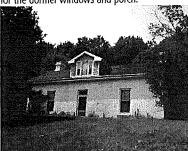
East elevation of the southern portion of the house; most likely the original façade was stone, the current stucco was applied later.
