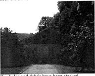
Hay bales and debris have been stacked against the wall of the north façade. Trees and plants shelter the space trapping moisture. Deterioration of the stuce has occurred along the lower portion behind the stack of debris and hay.
