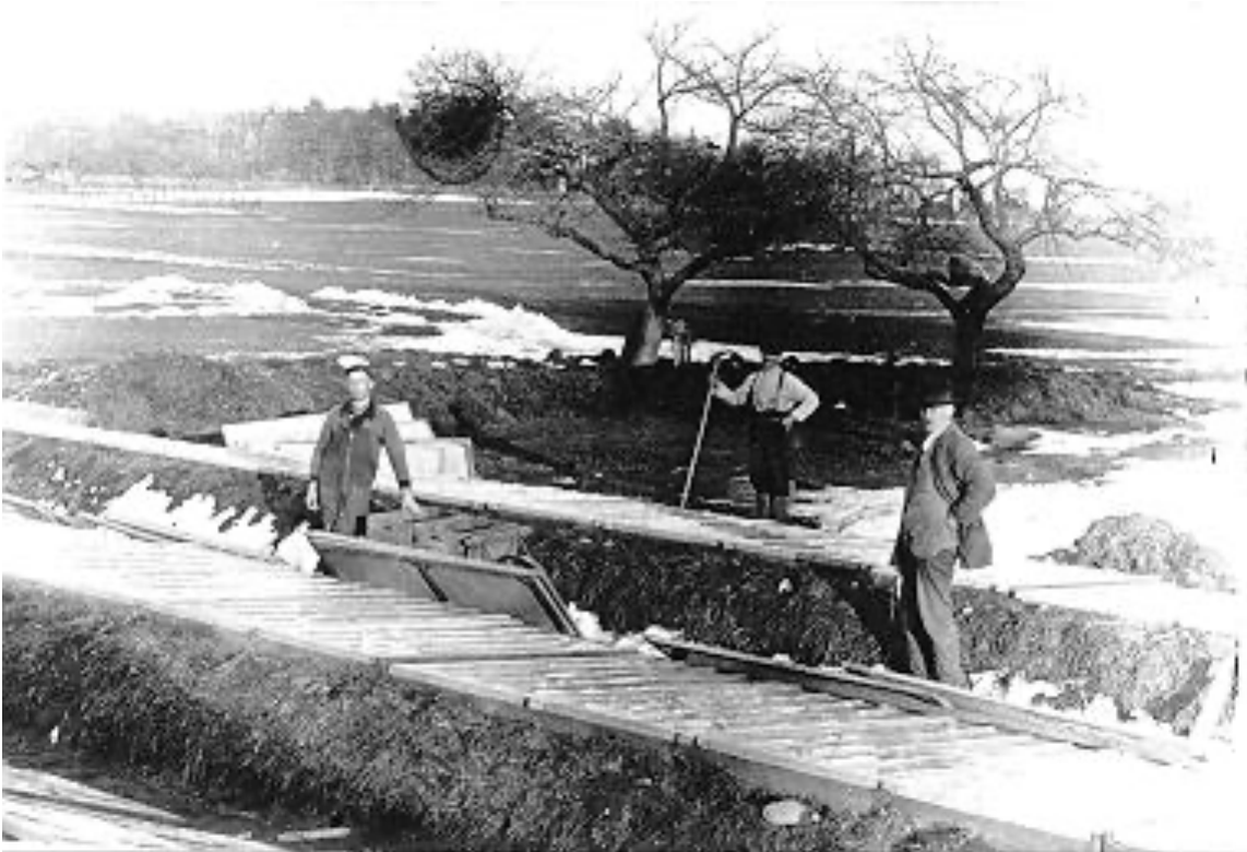
c.1897 PHOTO - George Unsworth's first cold frames built in the 1890s from sash from the Crystal Palace and erected in an old fruit orchard on his property BHS
