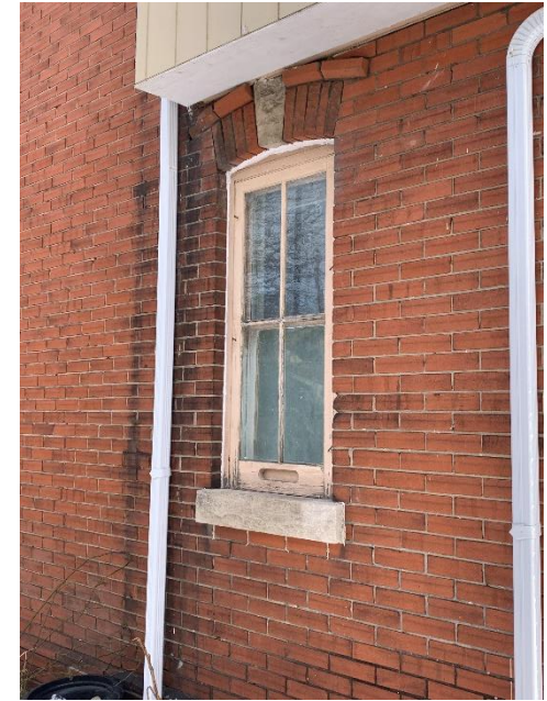
North elevation original wood window
