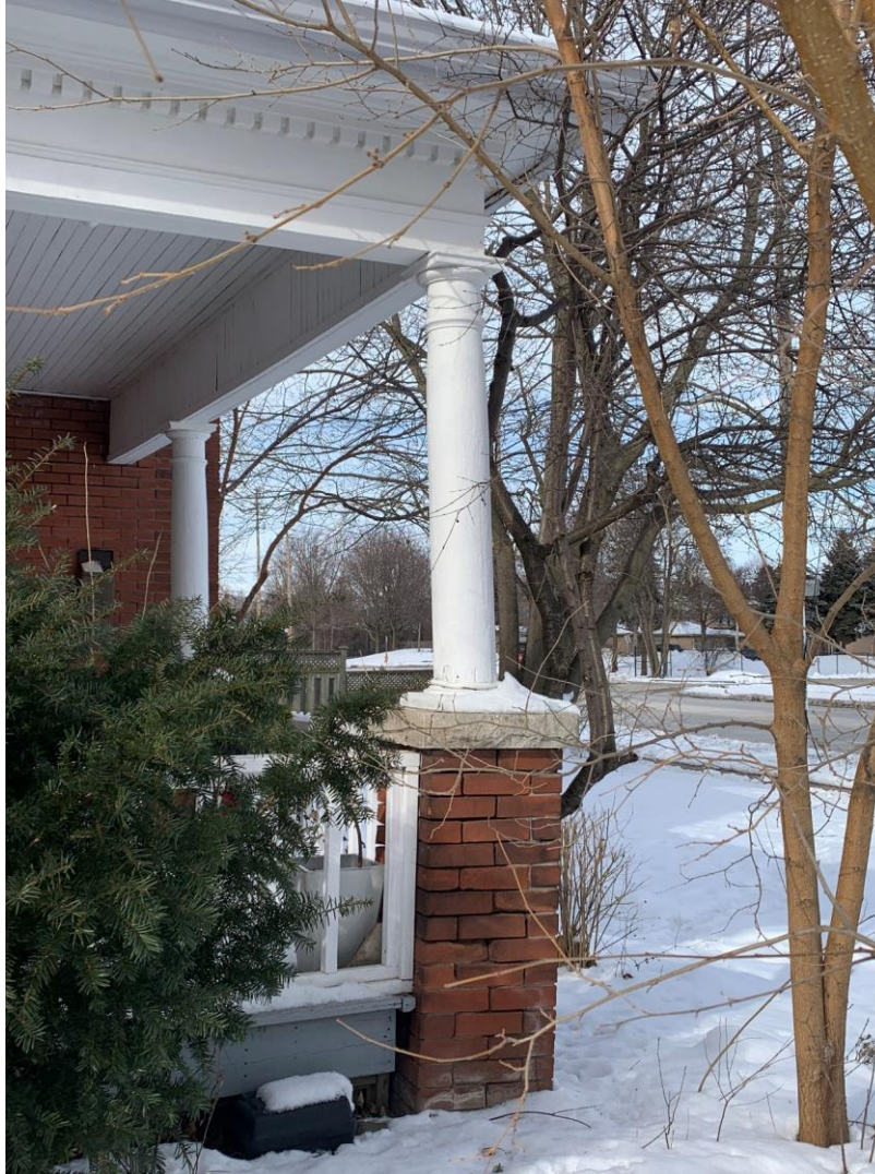
Front porch column buckling outward
