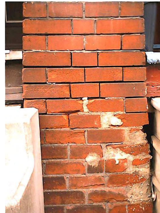
Progressive deterioration: The mortar was eroded due to rainwater splashing on the porch and steps. Failure to repair allowed more and more water into the masonry. The bricks below the failed mortar are now spalling and washing away. Neglect has turned a minor maintenance job into a major repair project.
