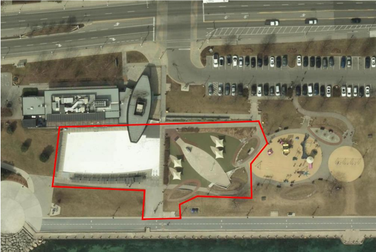
Aerial of the Waterfront Centre
