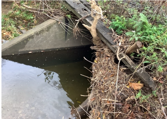
Upstream Structure Face (Photo)
