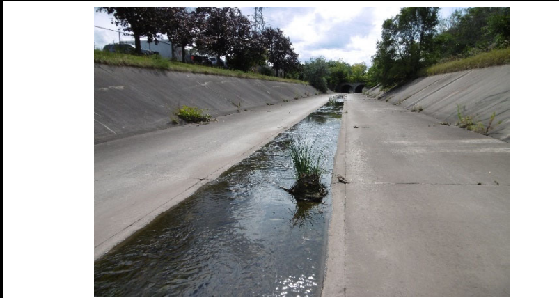
Watercourse Looking Upstream
