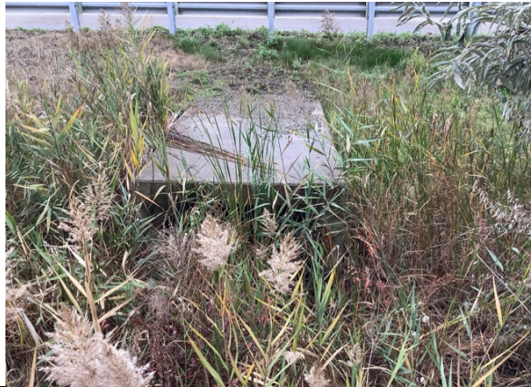
QEW Structure Face (Photo)
