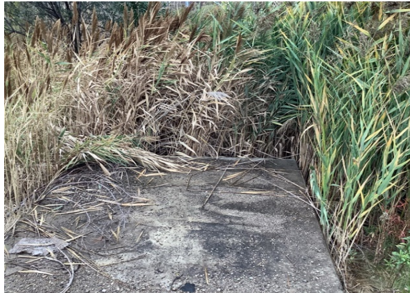
QEW Structure Face (Photo)
