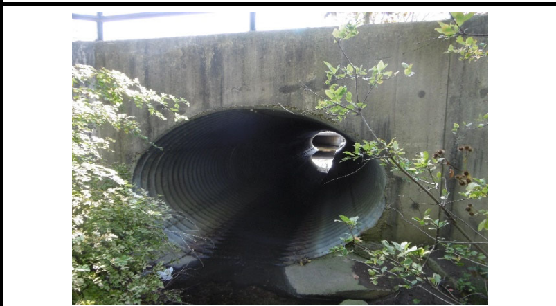
Upstream Structure Face (Photo)
