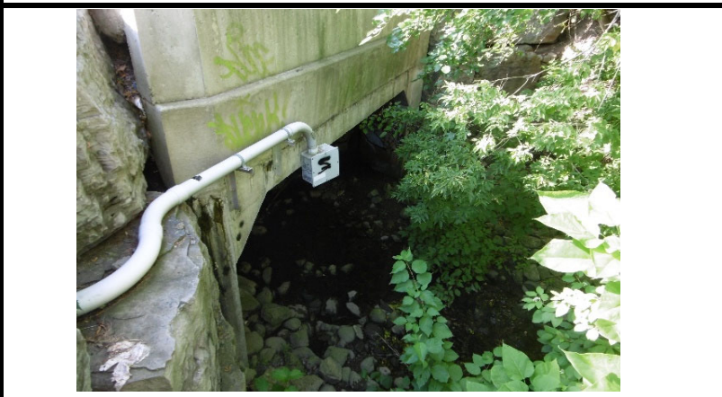
Upstream Structure Face (Photo)
