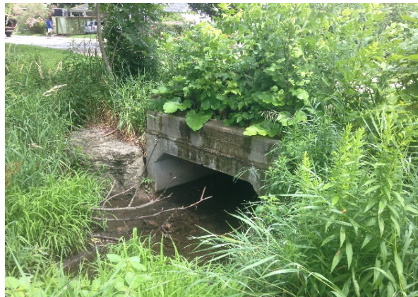
Upstream Structure Face (Photo)
