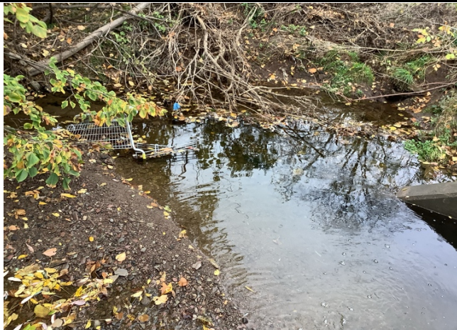
Watercourse Looking Upstream
