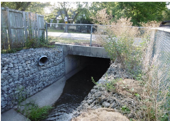
Upstream Structure Face (Photo)
