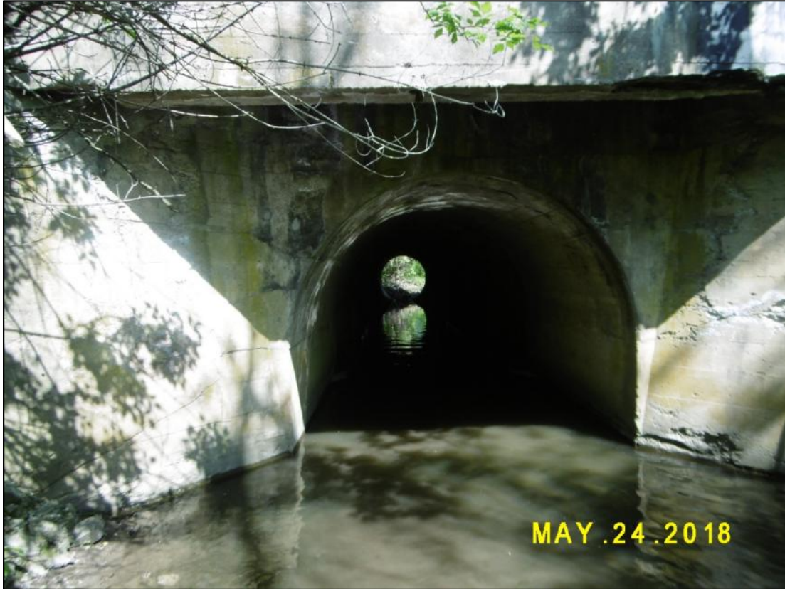
Photo 1 – Outlet – South Side
