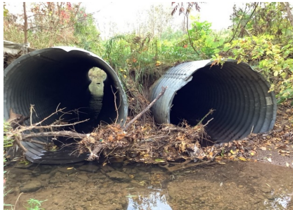
Upstream Structure Face (Photo)
