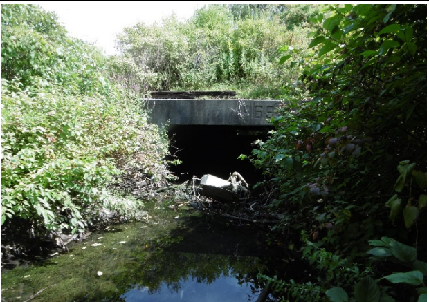
Upstream Structure Face (Photo)
