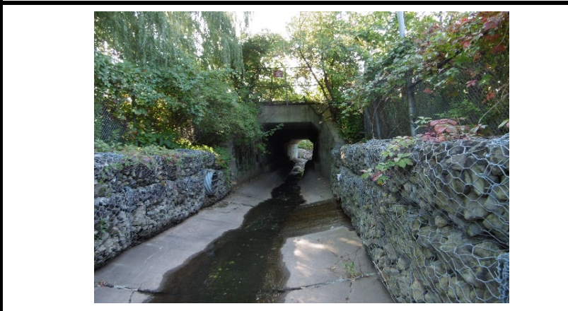
Upstream Structure Face (Photo)
