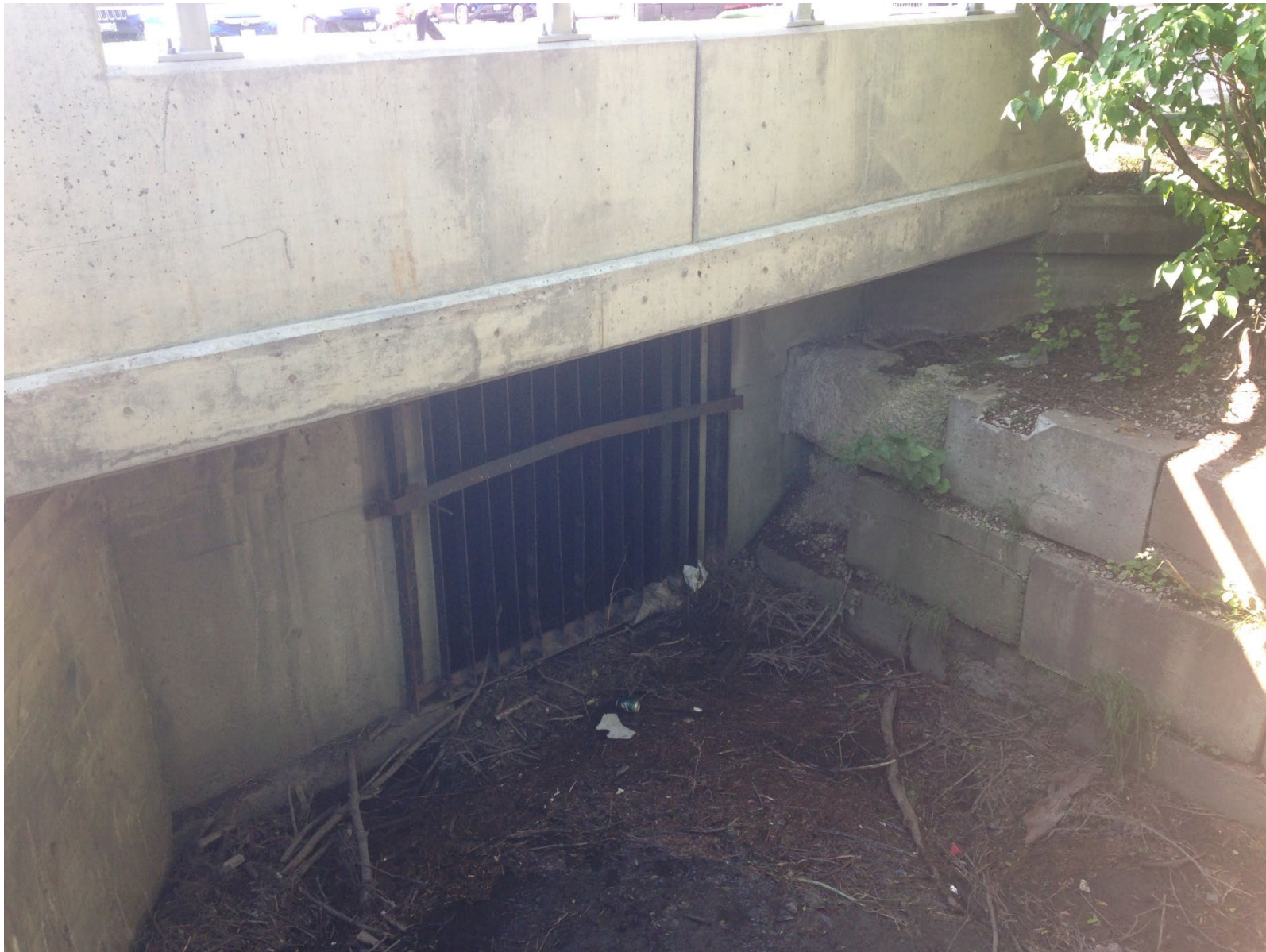
FIGURE E1: UPSTREAM FACE OF BLAIRHOLM AVENUE STORM SEWER ENCLOSURE
