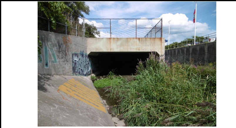
Upstream Structure Face (Photo)
