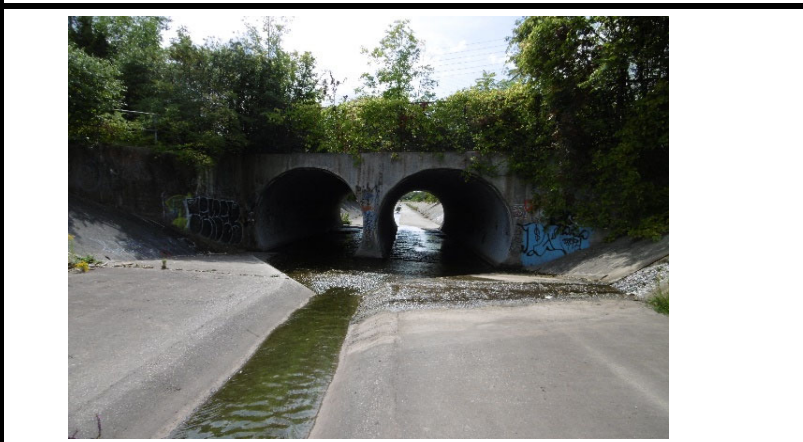
Upstream Structure Face (Photo)
