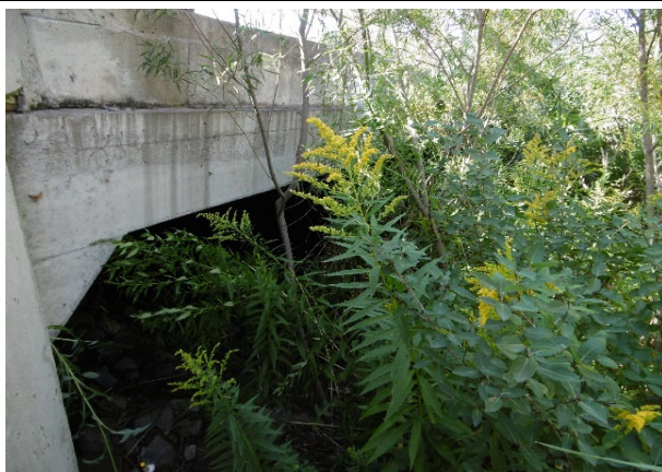
Upstream Structure Face (Photo)
