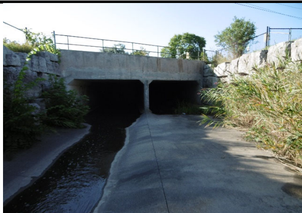
Upstream Structure Face (Photo)
