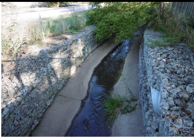
Watercourse Looking Upstream
