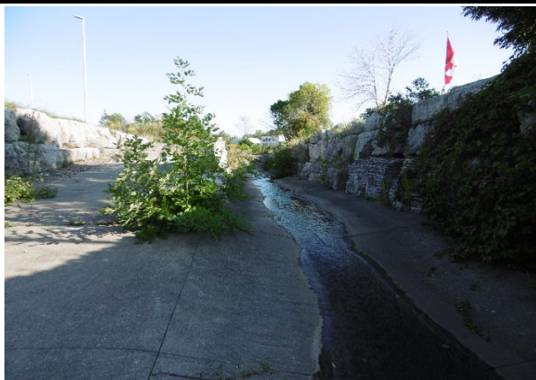
Watercourse Looking Upstream
