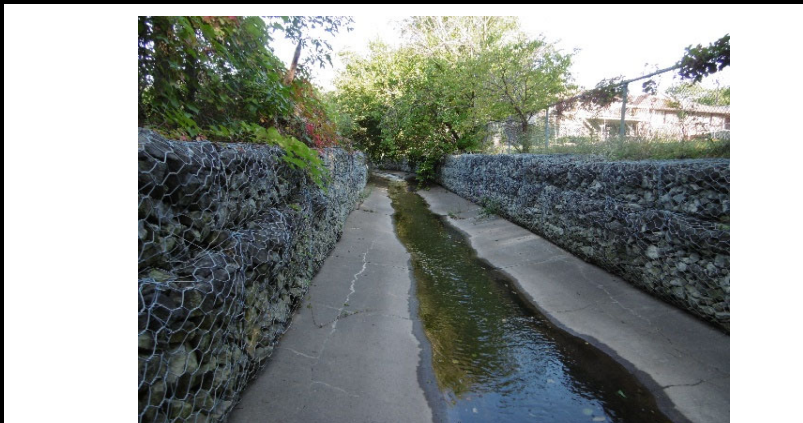
Watercourse Looking Upstream
