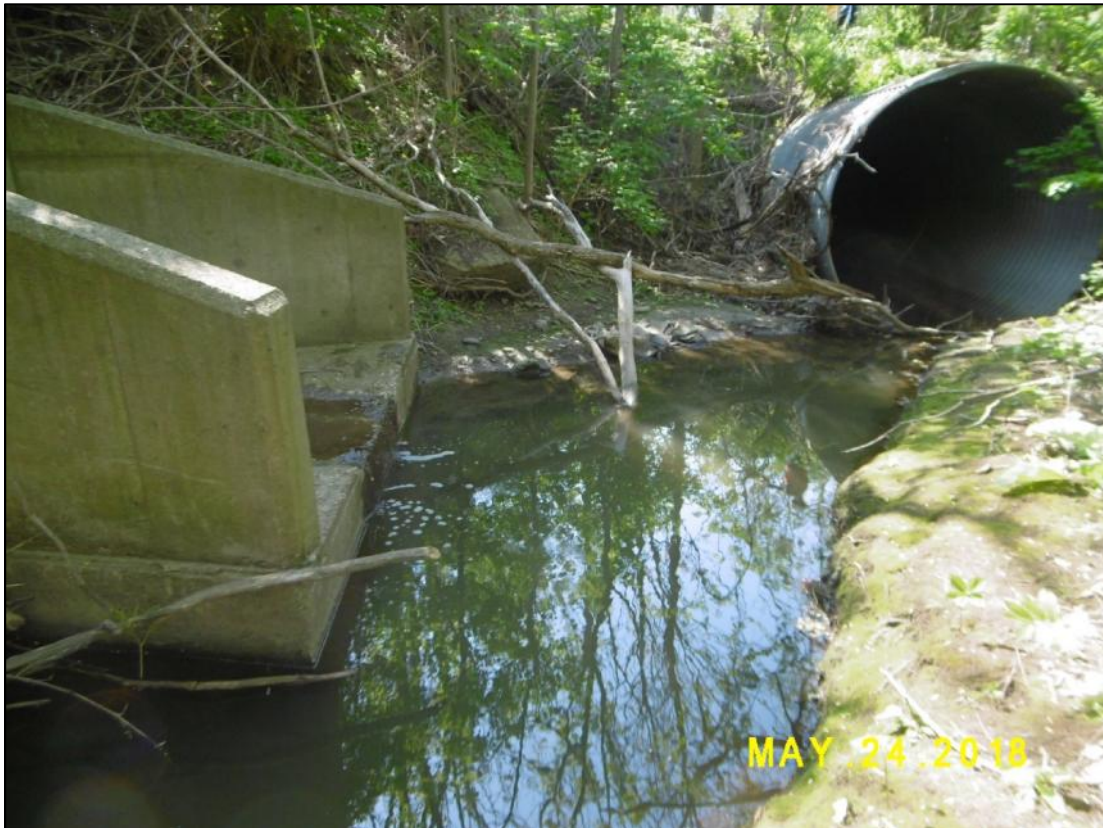
Photo 2 – Inlet & Storm Drain – North Side
