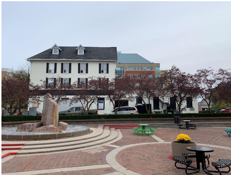
Photo of Side (North) Elevation defining the edge of Civic Square
