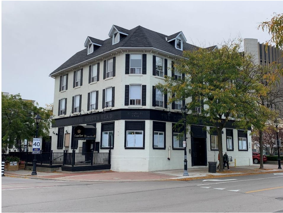
Photo of Chamfered corner and elevations facing Brant Street and Elgin Street
