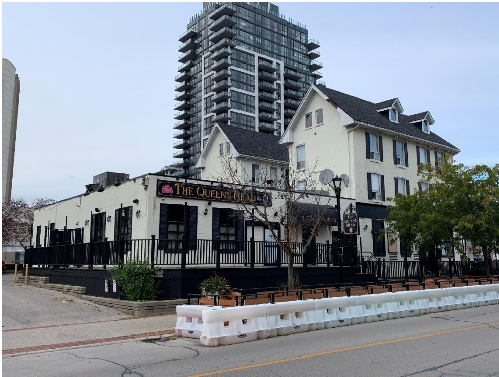
Photo of Rear (West) Elevation
