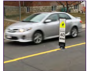
Flex Posts (Temporary)
