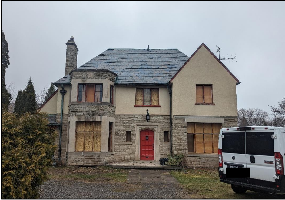
Figure 1: Front Elevation of Stone and Stucco Building
