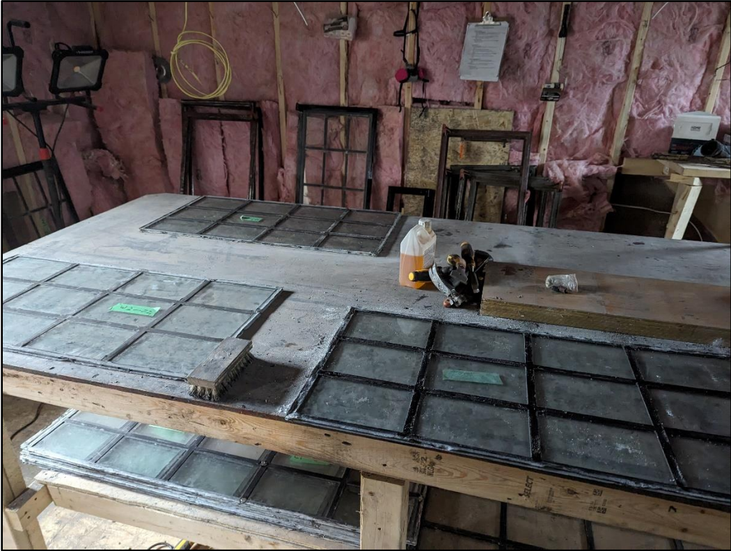
Figure 3: On-Site Restoration of Windows
