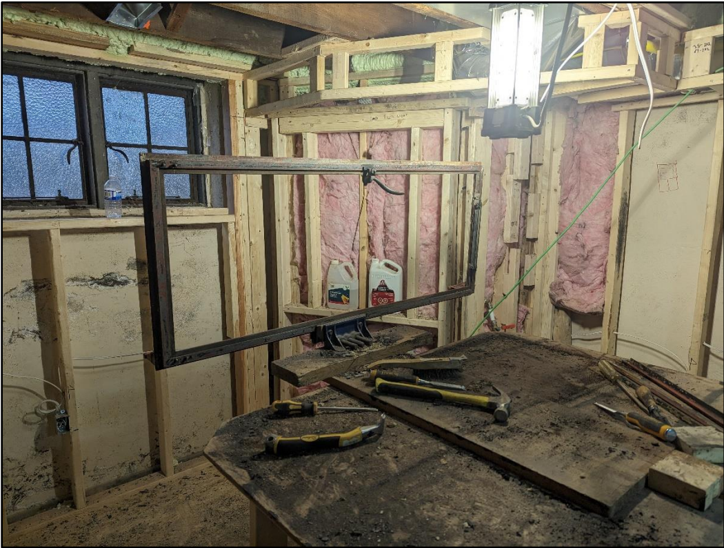
Figure 4: On-Site Restoration of Windows
