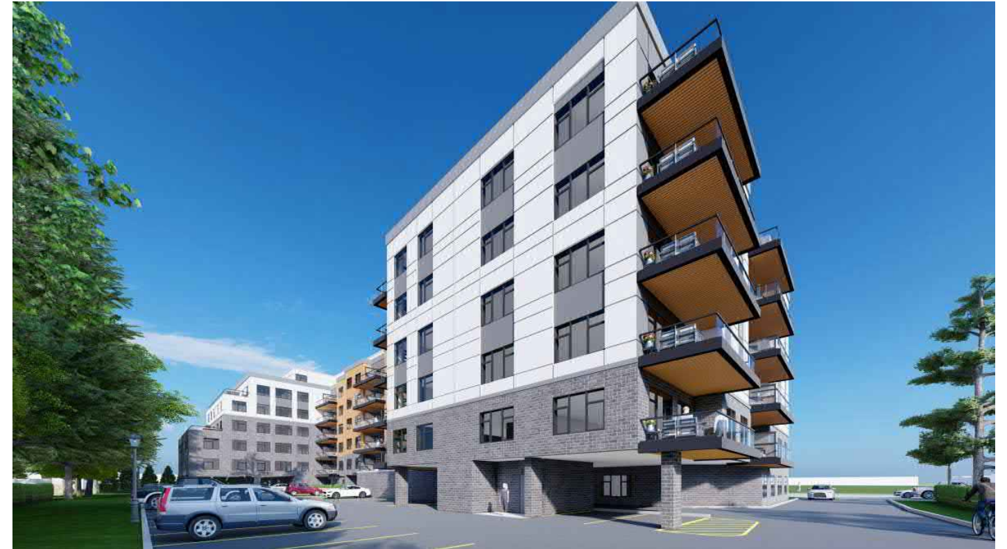
Back of Building
