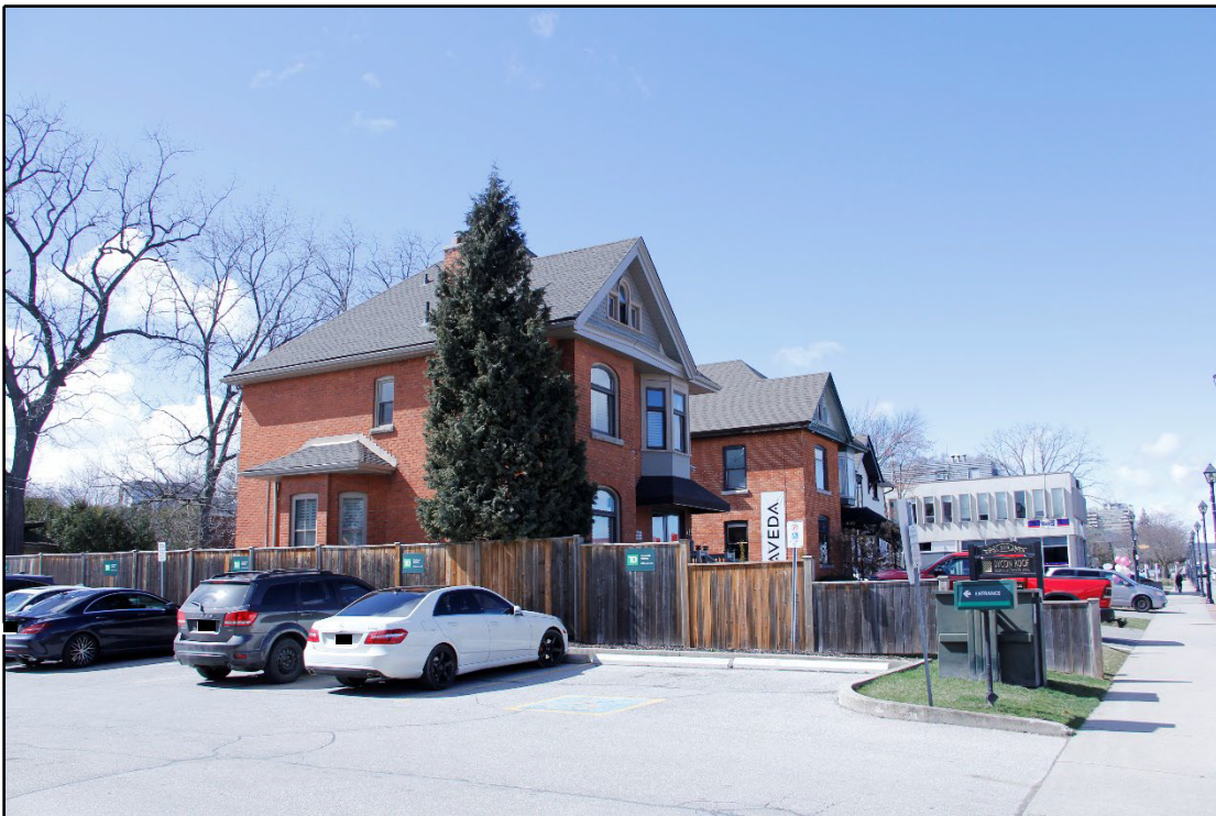
Figure 2: Side (South) Elevation of Brick Building
