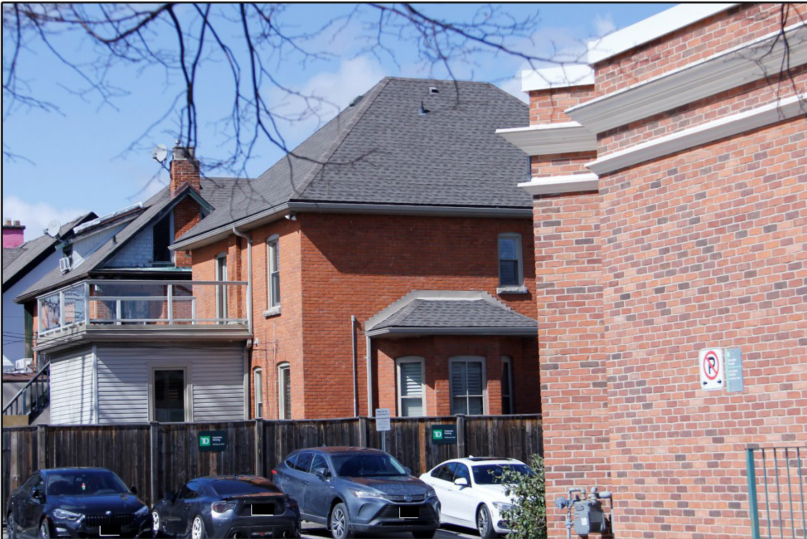
Figure 4: Rear Addition, Rear Elevation and Side (South) Elevation of Brick Building, as Seen from Caroline Street to the South
