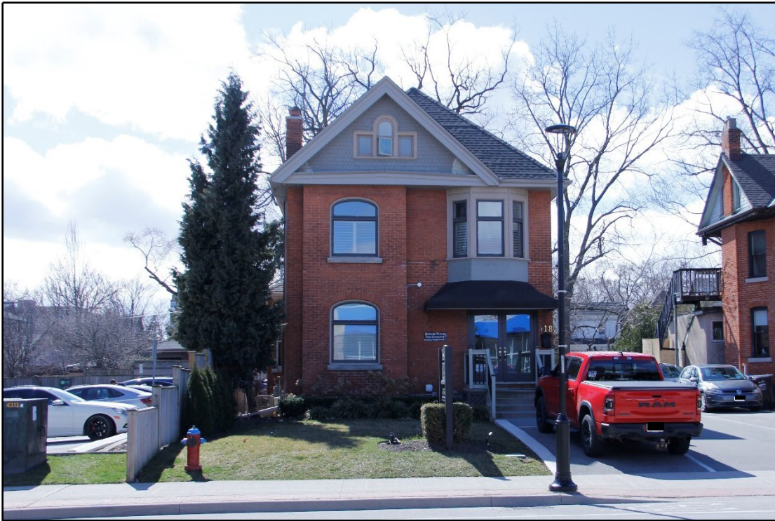
Figure 1: Front Elevation of Brick Building
