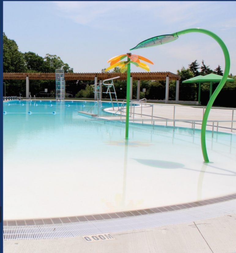
Mountainside and Nelson Pool Renovation
