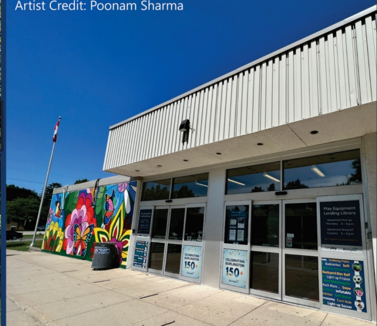
Aging infrastructure requires renewal, replacement or repurposing
