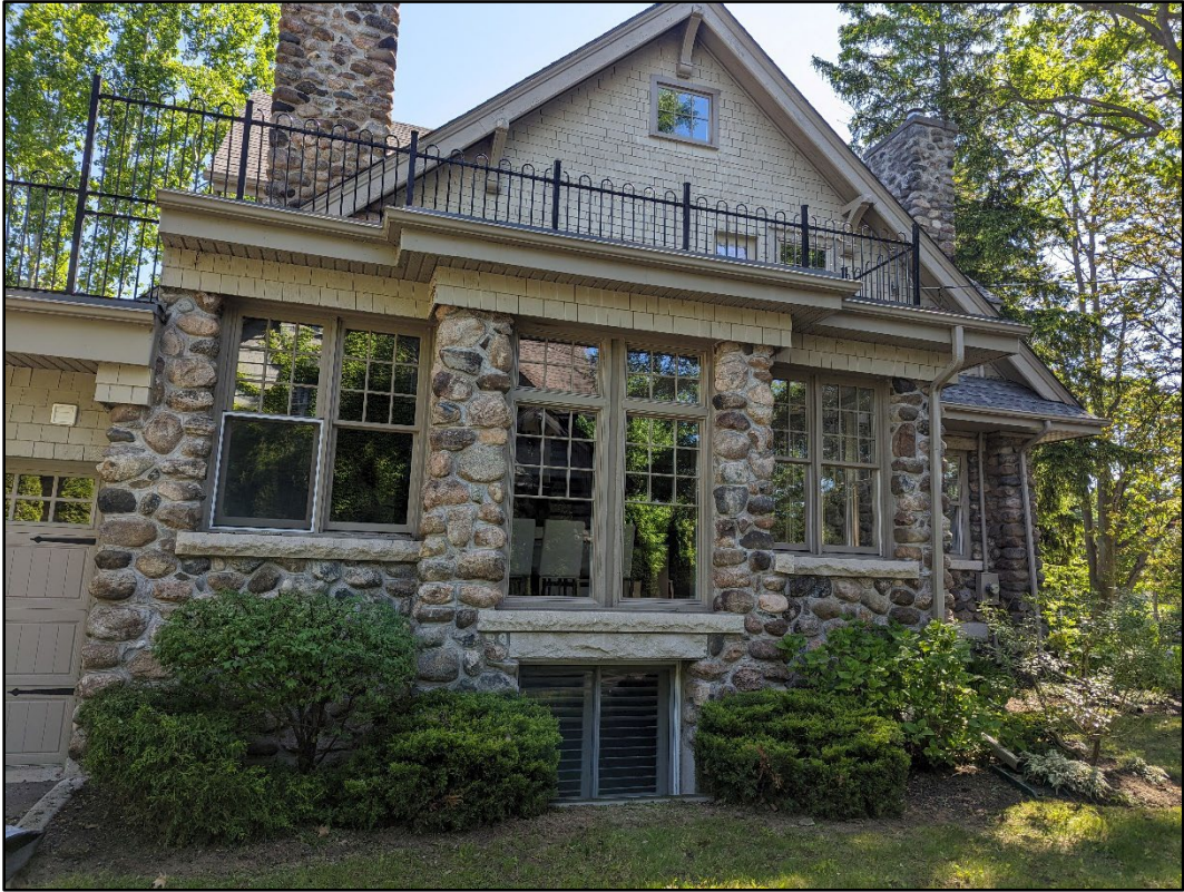
Figure 3: Side (West) Elevation of Subject Building
