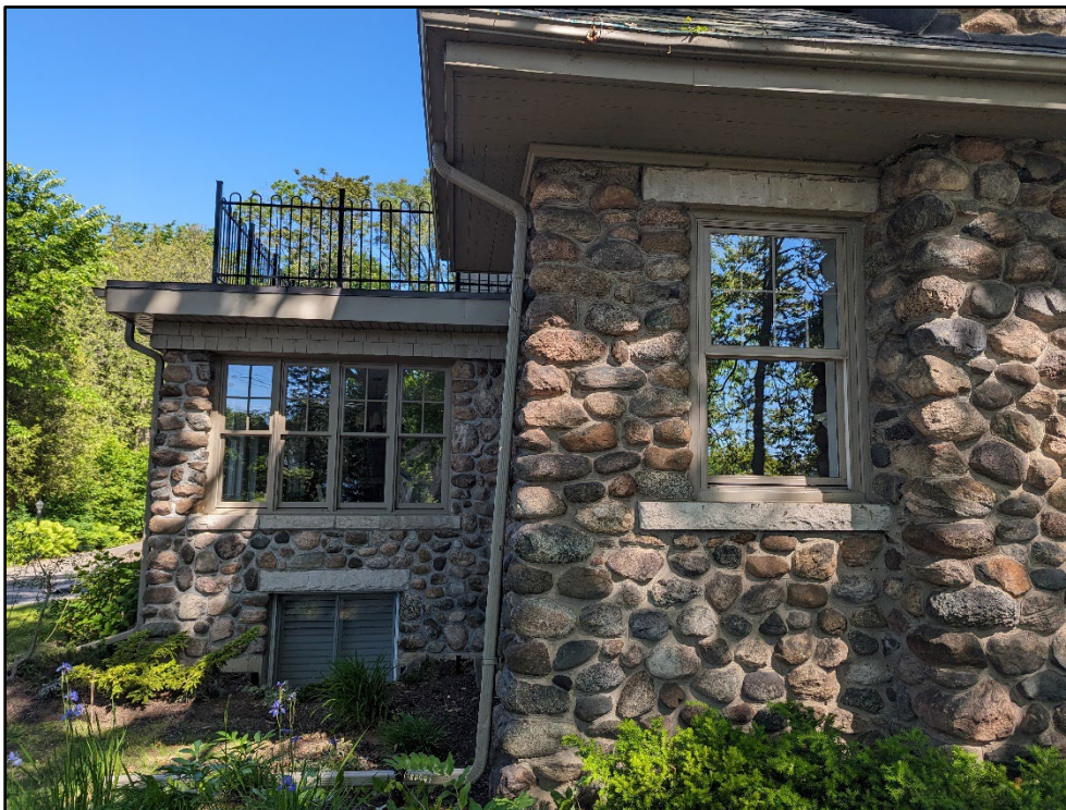
Figure 2: West Portion of Front Elevation
