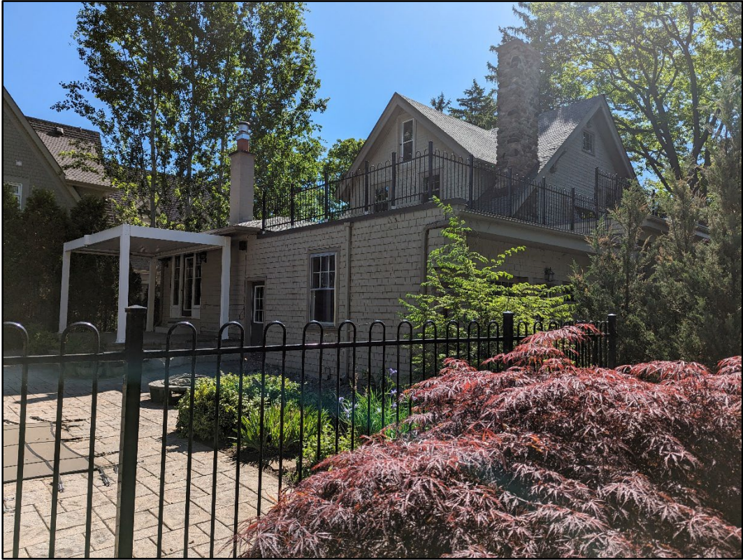
Figure 5: Northwest Corner of Single-Storey Rear Addition
