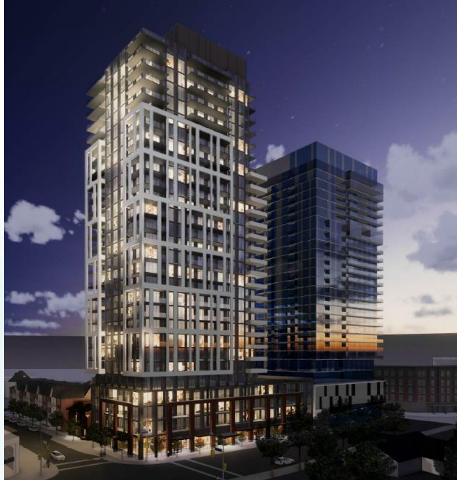
2069 Lakeshore Rd. and 383 Pearl St Under Construction 291 residential units
