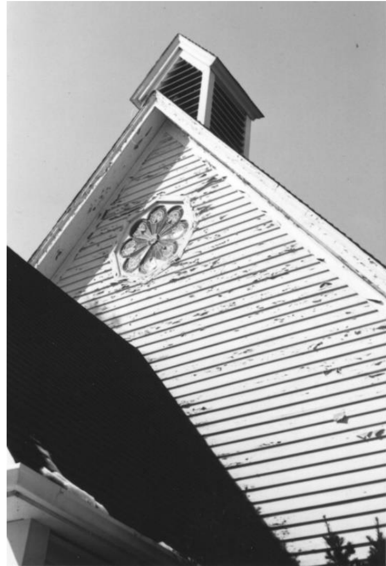
Figure 194: The front (south) façade of St. Luke's showing the state of the wood siding before it was covered with aluminum siding [Burlington Historical Society].
