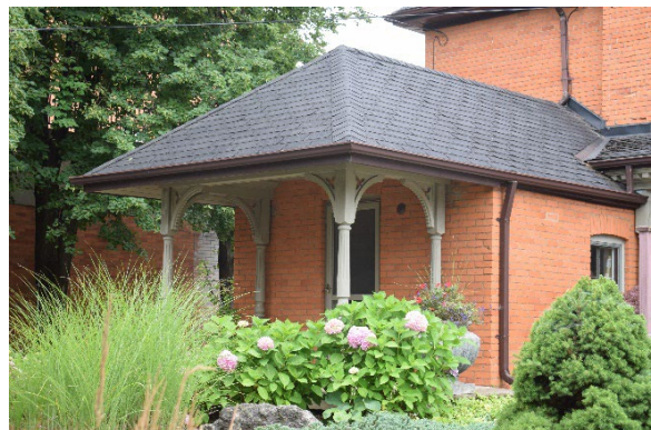
Photo 3.10: Rear porch with porch brackets and posts, looking southwest
