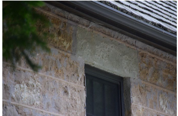
Photo 3.8: Stone lintel above window, looking southwest
