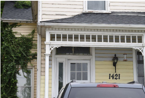
Photo 3.7: Front door with transom and sidelight, looking northeast
