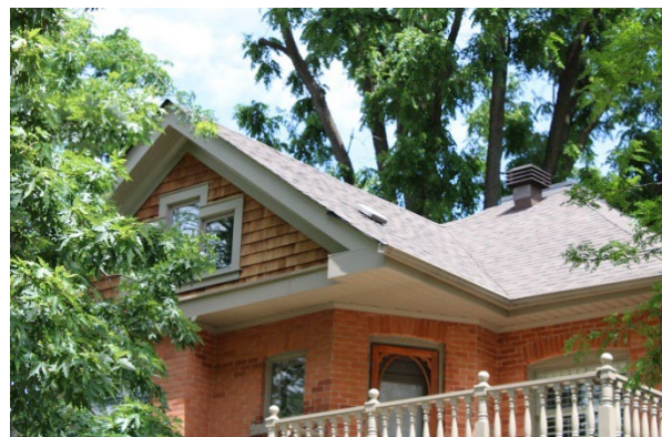
Photo 3.6: Wood shingles on the front gable, looking northeast
