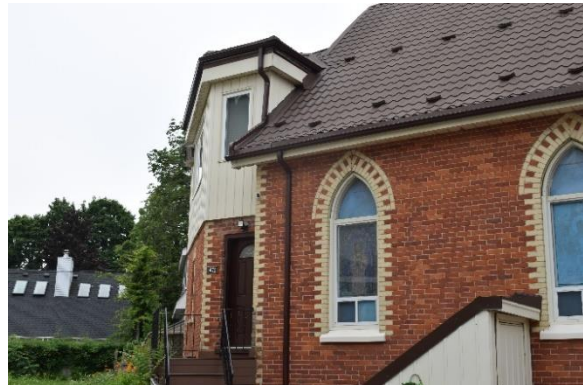
Photo 3.8 Original one-storey rear component and 20 th century addition with vinyl siding.
