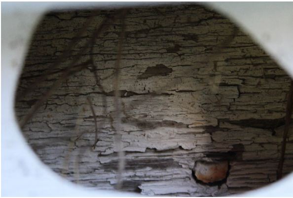
Photo 5: Wood siding visible underneath vinyl siding on west elevation, looking northeast
