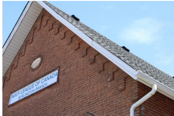
Photo 3.8 Brick corbels, looking north
