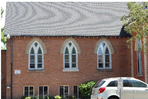
Photo 3.10 Pointed arch windows with buff brick hood molds, looking east
