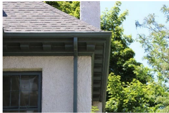
Photo 3.8: Dentil detail, looking west
