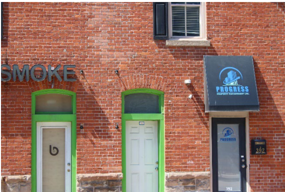
Photo 3.7 Representative of brick voussoirs, looking west
