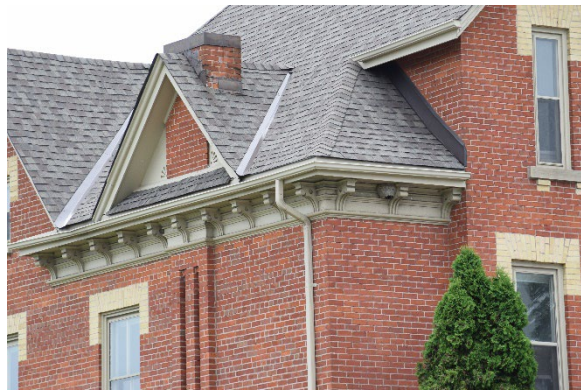
Photo 3.10: Frieze and brackets along roofline, looking southwest.
