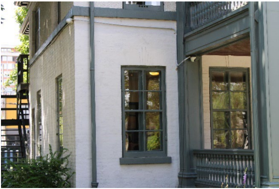
Photo 3.5: Wood sash window detail, looking southwest
