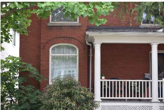
Photo 3.5: Arched window with brick voussoirs, looking southwest
