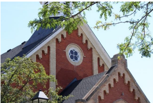
Photo 3.3 Buff brick detailing on gable peaks, looking southeast
