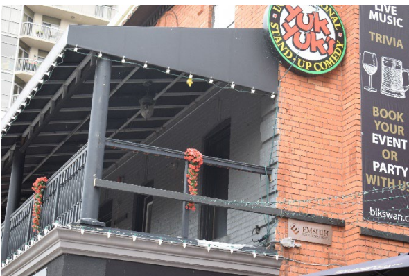
Photo 3.9: Brick quoins along the front façade of building, looking southwest
