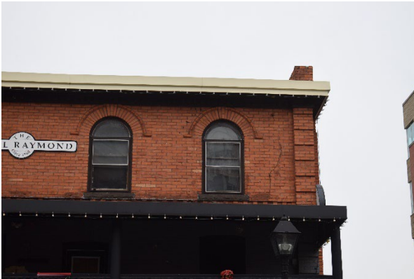
Photo 3.5: Third storey windows with drip moulds, looking northwest
