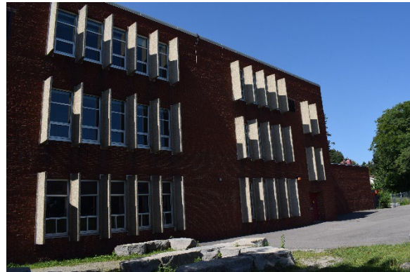
Photo 3.21: Concrete window fins detail, on northeast façade 1965 addition, looking northwest
