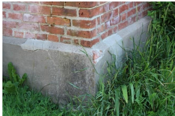
Photo 3.10 Signs of a red brick foundation covered by concrete parging, looking east
