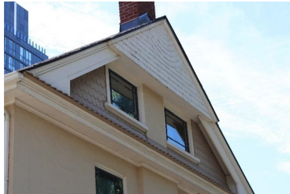
Photo 3.8 Shingle detail on north gable peak, looking south
