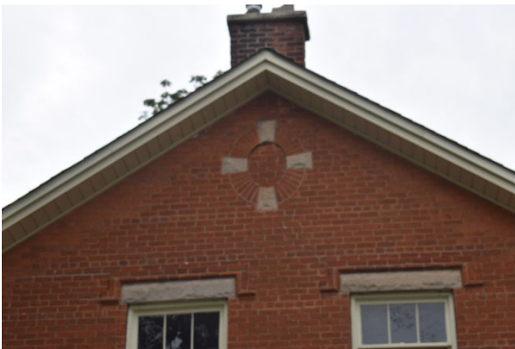
Photo 3.10: Bricked-in ocular window on east façade, looking west
