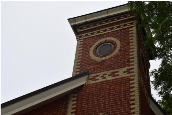
Photo 3.7 Dichromatic brick ringed oculus window, chevron pattern, brick dental moulding, and brick quoins.
