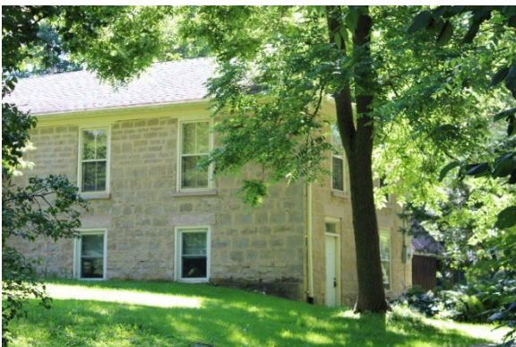
Photo 3.5: West façade, with stone lintels and concrete sills, looking southeast.
