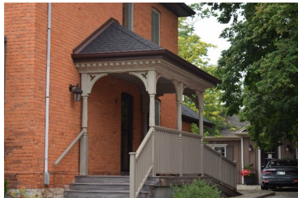
Photo 3.8: Side porch with dental trim and porch brackets and posts, looking north
