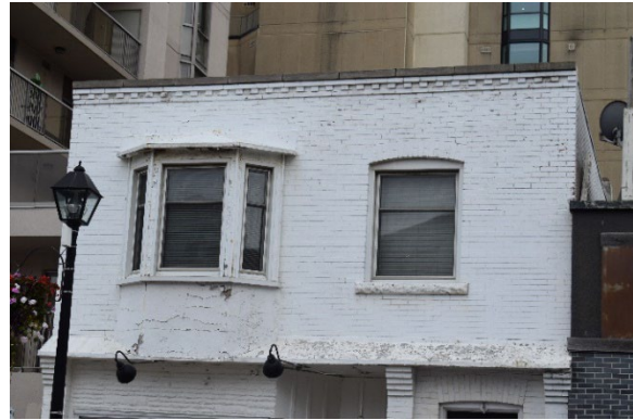
Photo 3.4: Second storey bay window and window with painted brick voussoir and stone sill
