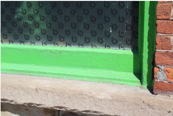
Photo 3.5 Representative detail of wood frame windows
