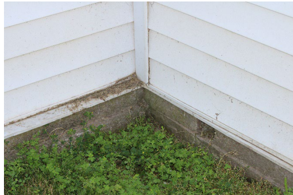
Photo 11: Parged concrete foundation detail on west elevation, looking east
