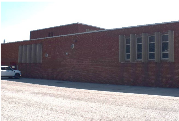
Photo 3.22: Concrete window fins detail, west façade, 1965 addition, looking east
