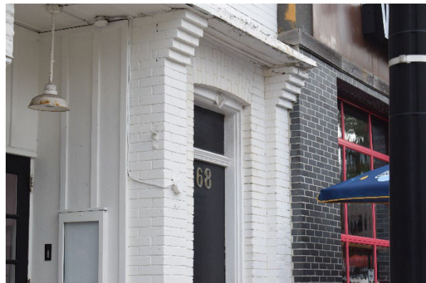
Photo 3.6: Secondary apartment entrance with transom, painted brick voussoir and stepped brick
