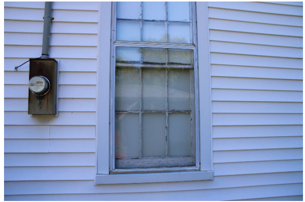
Photo 6: Wood sash windows with storm window detail on west elevation, looking east
