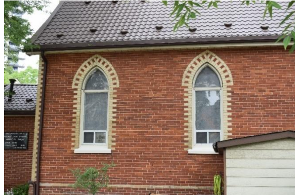
Photo 3.6 Windows with dichromatic brick dentilated trim and brick quoins.
