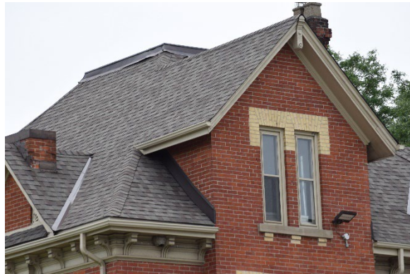
Photo 3.8: Projecting gabled wall dormer on north façade, looking southwest.
