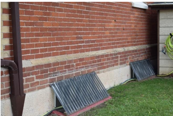
Photo 3.9 Parged foundation of original church building.
