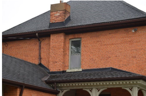
Photo 3.12: Brick voussoirs over windows and stone sill, looking southwest
