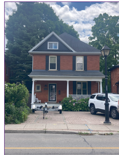
Street view of 1414 Ontario St.
