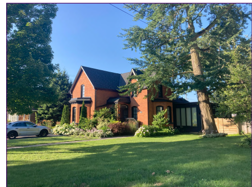
Street view of 460 Burlington Ave.
