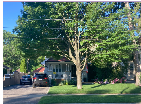
Street view of 426 Burlington Ave.
