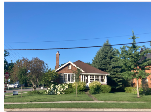
Street view of 454 Burlington Ave.
