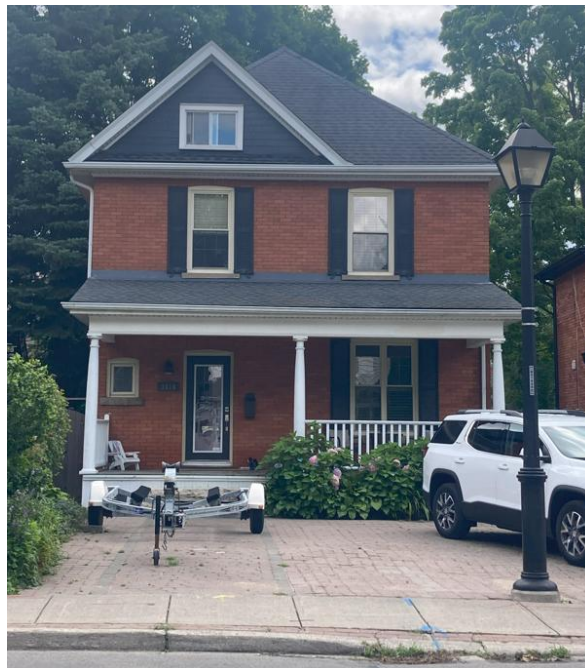
Figure 50 John Foster House, 1414 Ontario Street. An example in Burlington Stripped Edwardian Classicism.
