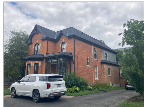
Street view of 437 Burlington Ave.
