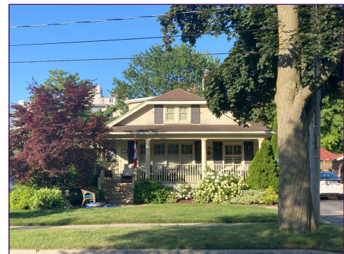
Street view of 422 Burlington Ave.
