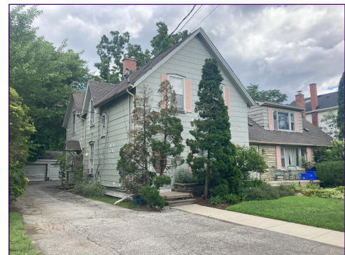
Street view of 419 Burlington Ave.
