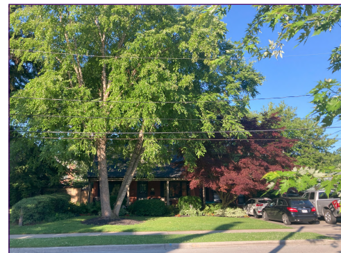
Street view of 436 Burlington Ave.
