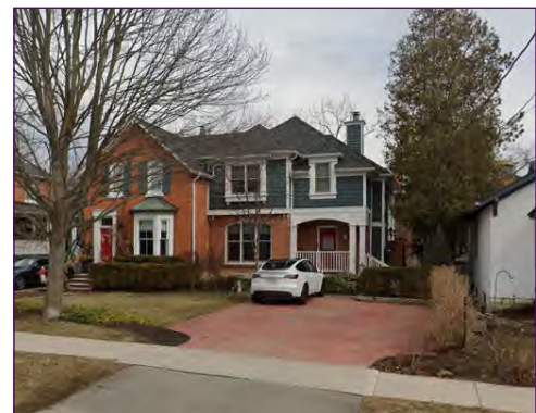
Street view of 457 Burlington Ave.
