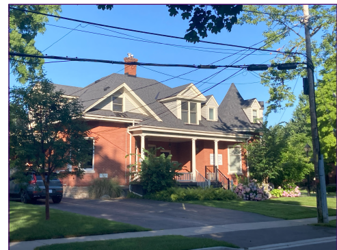
Street view of 482 Burlington Ave.
