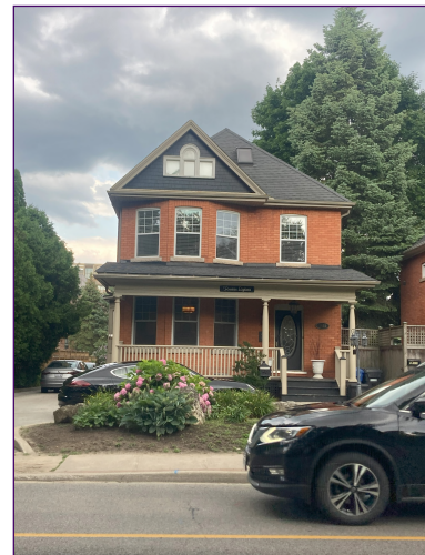
Street view of 1418 Ontario St.
