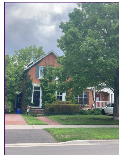
Street view of 461 Burlington Ave.
