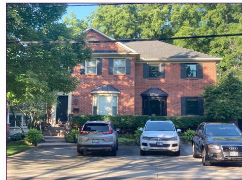
Street view of 476 Burlington Ave.
