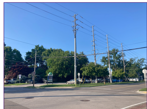
Street view of 446 Burlington Ave.
