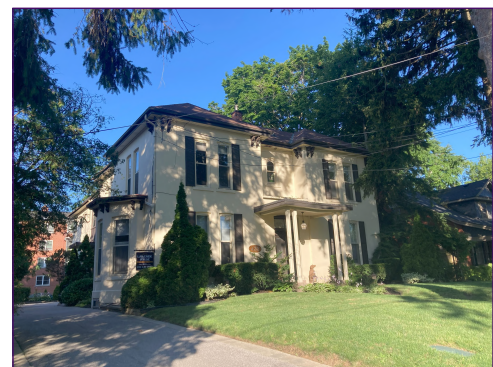
Street view of 432 Burlington Ave.
