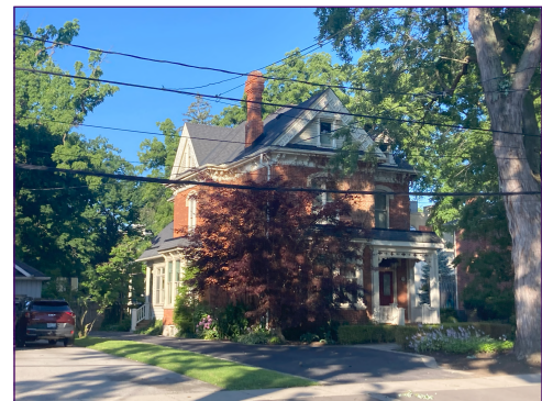
Street view of 472 Burlington Ave.
