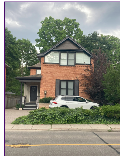
Street view of 1410 Ontario St.
