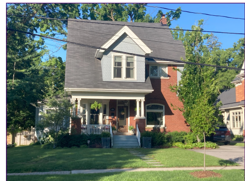
Street view of 466 Burlington Ave.
