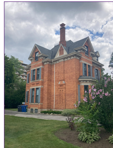
Street view of 431 Burlington Ave.
