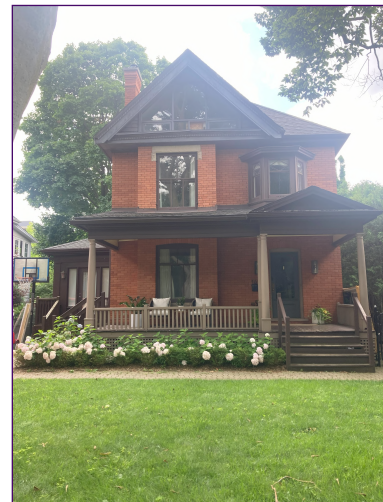
Street view of 1422 Ontario St.
