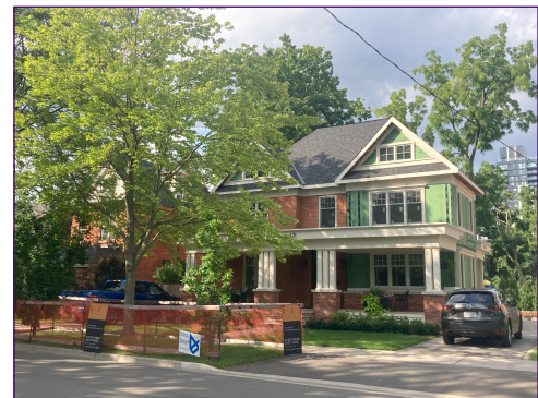
Street view of 471 Burlington Ave.
