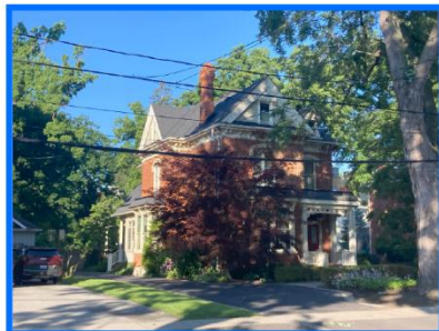
4 Looking towards 472 Burlington Ave.
