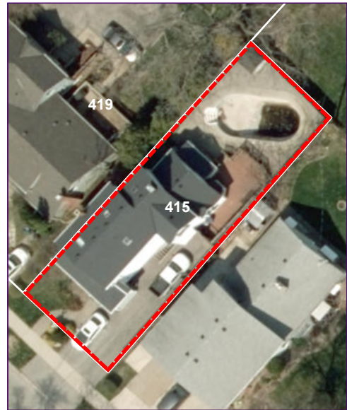
Aerial view of 415 Burlington Ave.
