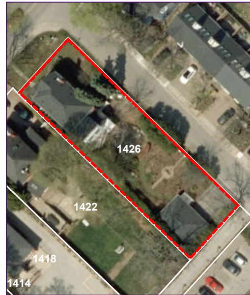
Aerial view of 1426 Ontario St.
