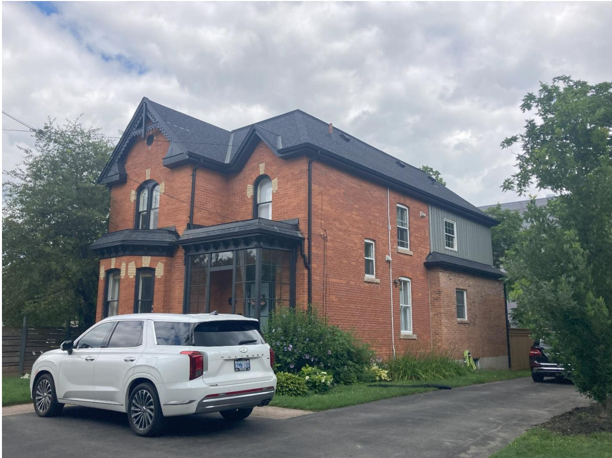
Figure 3.25: Addition at the rear of 437 Burlington Avenue.
