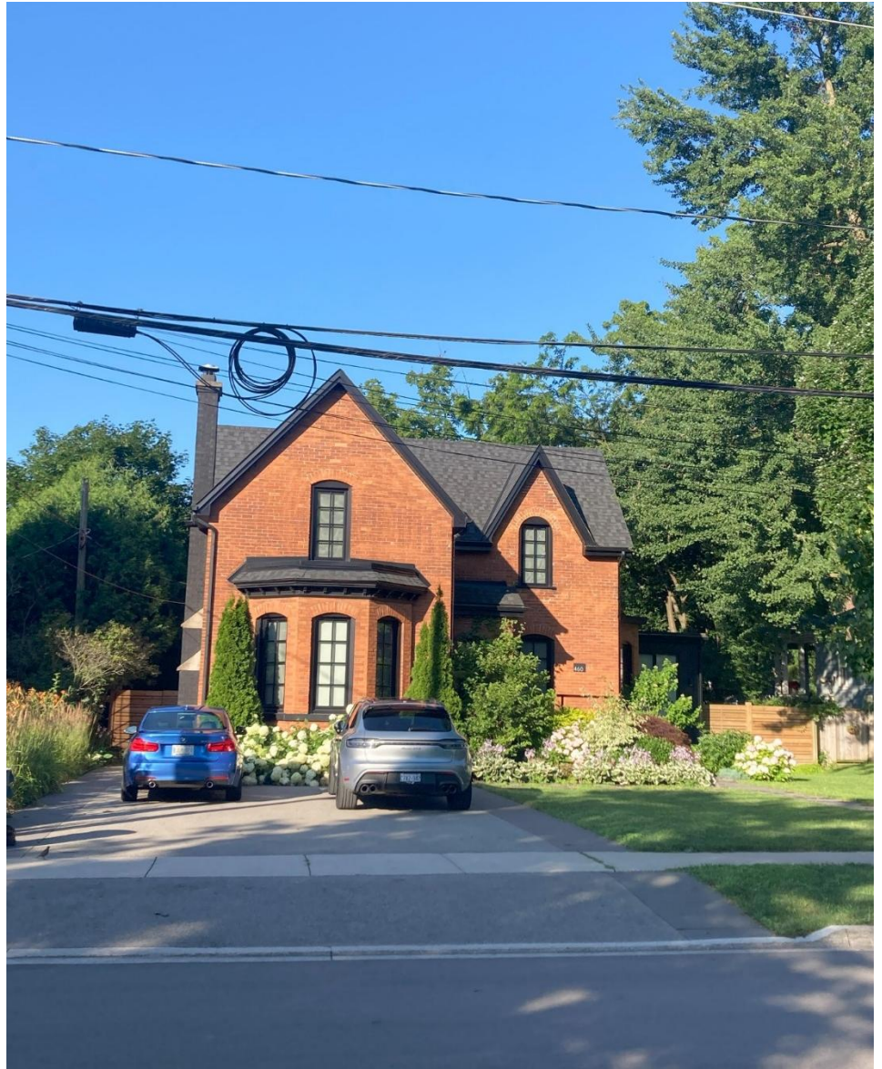
Figure 3.11: An example of complimentary modern wood fencing at 460 Burlington Avenue.
