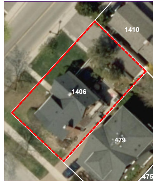
Aerial view of 1406 Ontario St.
