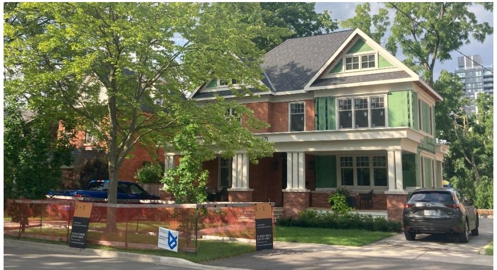
Figure 3.20: Image of an excellent example of an addition respecting the massing, window line, porch and roofline of the existing building at 471 Burlington Avenue.
