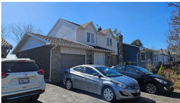
Existing garage (and location of proposed addition)
