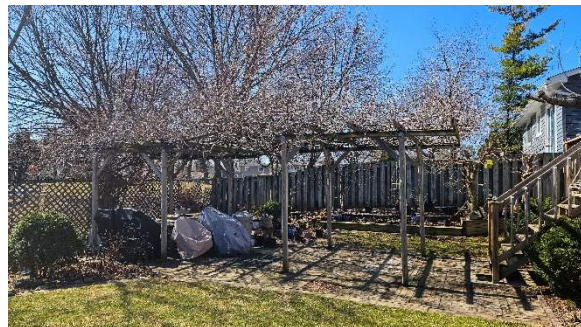
Existing accessory structure
