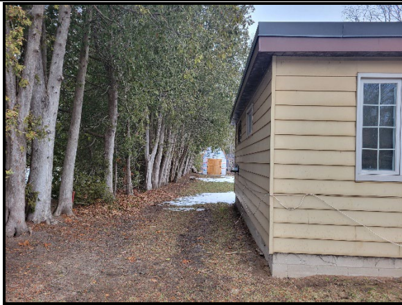
View of the northwesterly corner
