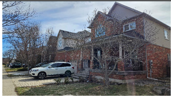
View of front and side yard, at covered porch
