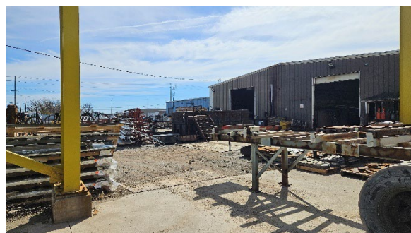
Rear yard of subject property (approximate location of proposed addition)
