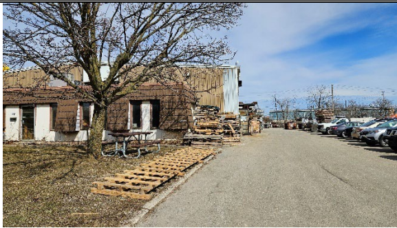
Front view of subject property at south entrance
