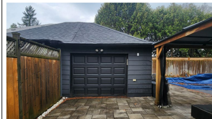
View of existing accessory building in south yard.
