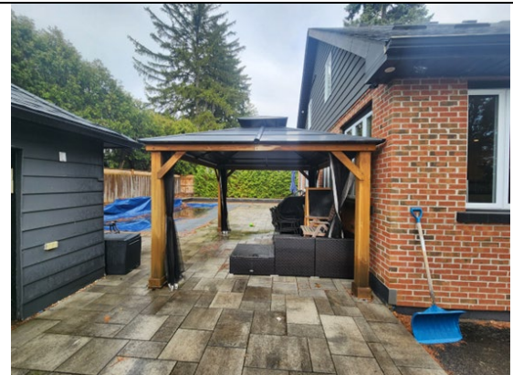
View of rear yard and accessory structure (pergola).
